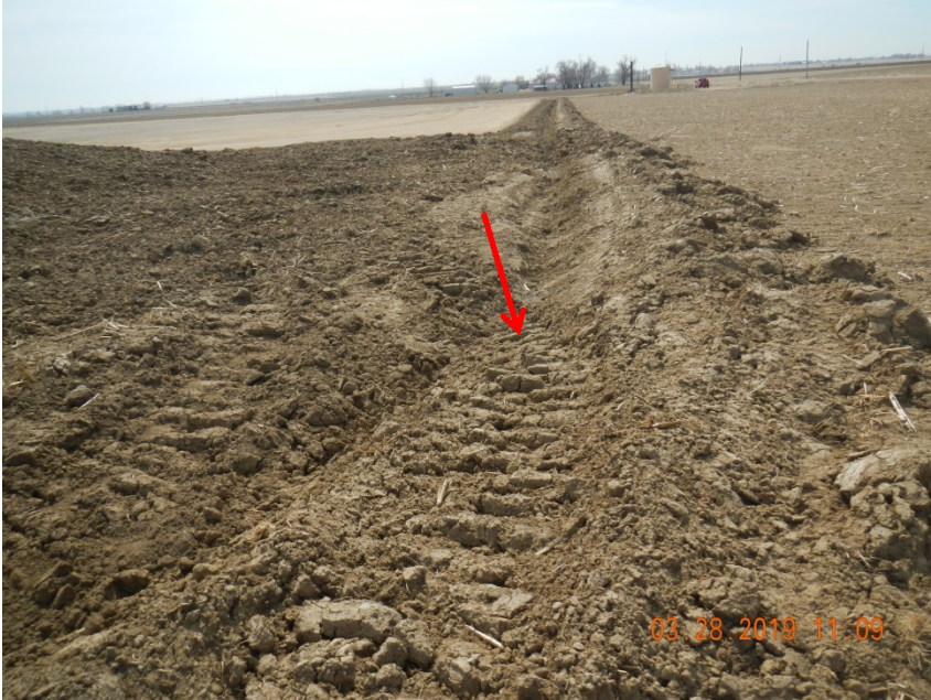
Photo 5. Photo taken from the northwestern perimeter of the location, facing South. Photo illustrates the ditch and berm BMP that has been installed around the perimeter of the location has been tracked through by equipment.
