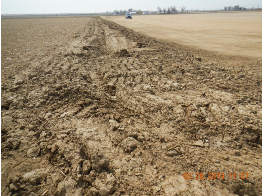
Photo 1. Photo taken from the northeastern perimeter of the location, facing South. Photo illustrates a ditch and berm BMP that has been installed around the perimeter of the location. However, the ditch and berm BMP is not compacted in several areas along the perimeter.
