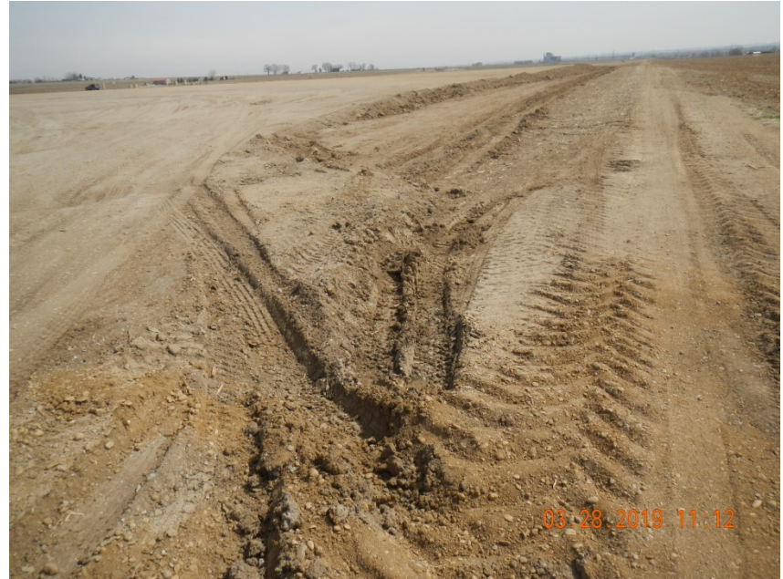
Photo 8. Photo taken from the southwestern perimeter of the location, facing South. No sediment traps with stabilized outlets were observed on location during construction.
