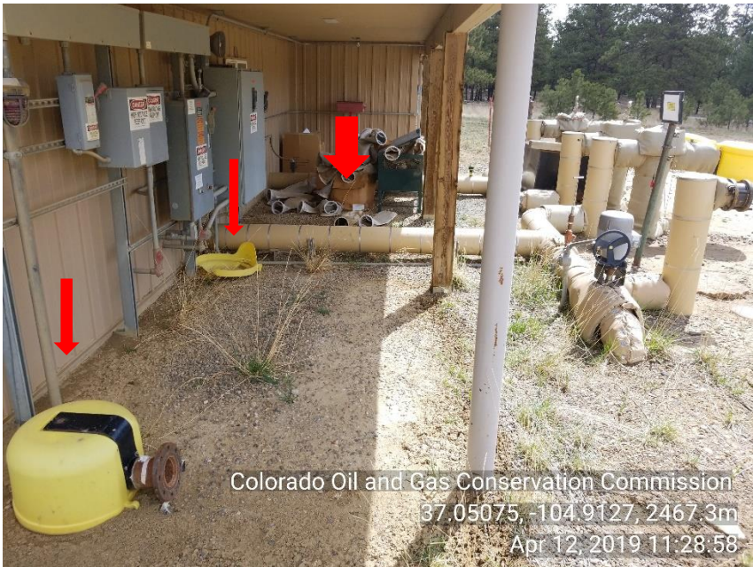
Photo 7 House Keeping What appears to be used filter pot filters laying on ground and unused unloading spill container.
