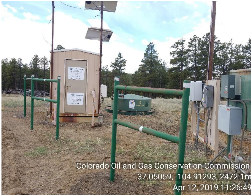
Photo 1 Duel Sep/meter house for HR#29-14 and HR#29-14V, 15bbl produced water tank and electric panel.
