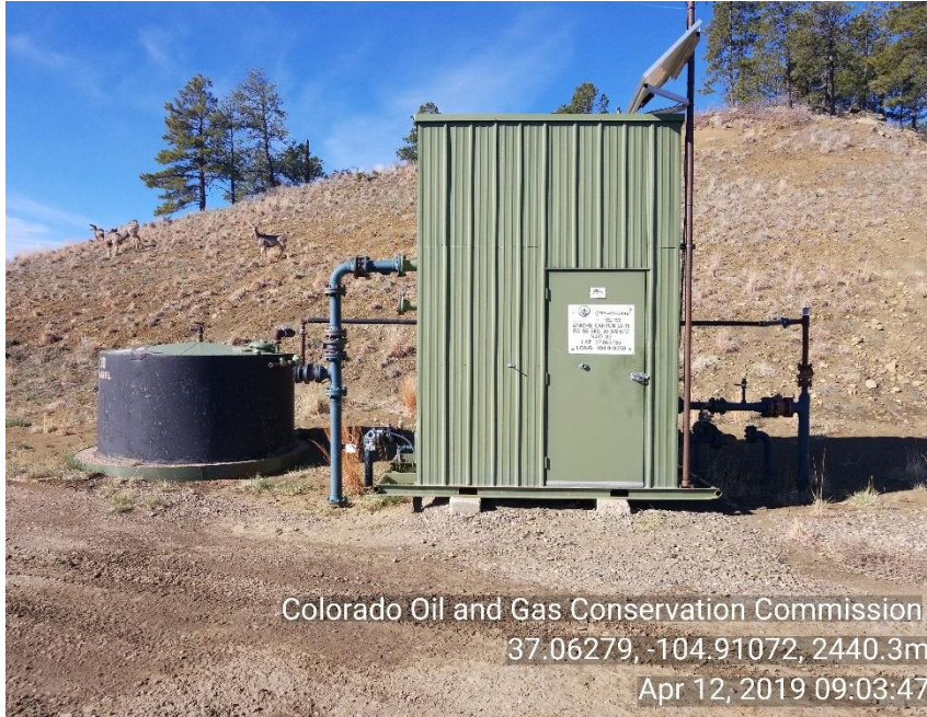
Photo 1 Sep/meter house . 30bbl produced water tank
