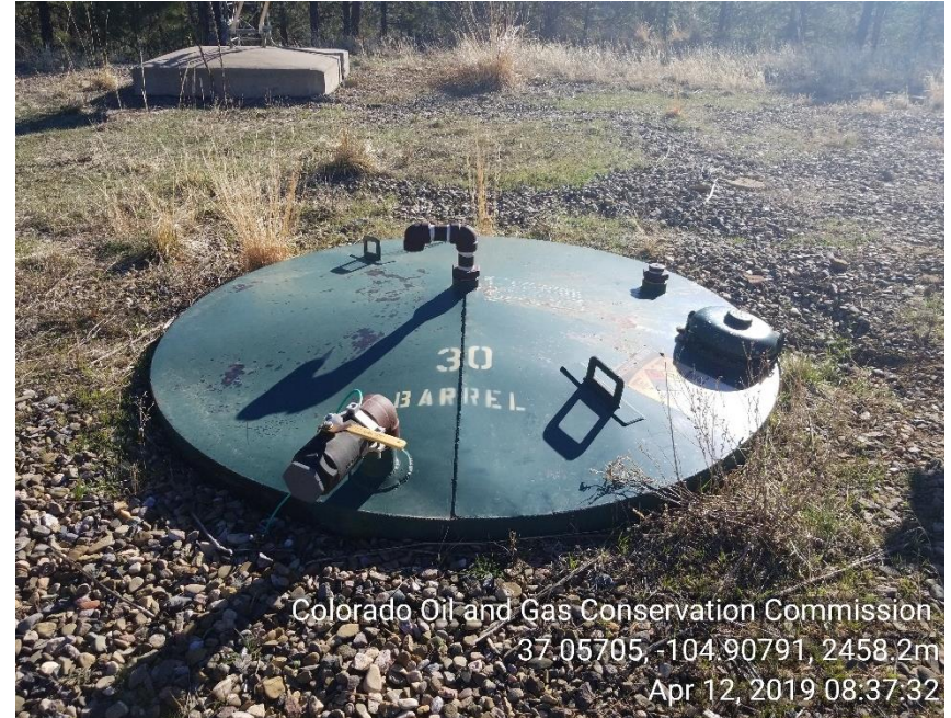
Photo 2 30bbl produced water tank
