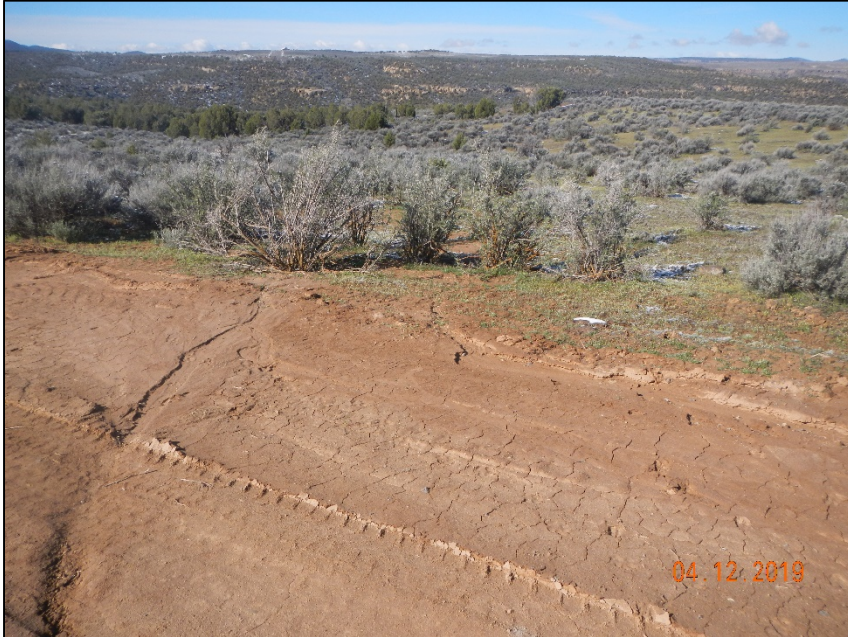
No BMP in place or maintained to keep erosion from leaving access road.
