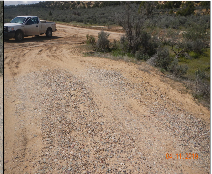
Evidence of erosion moving soil and storm water off the west side edge of location at the entrance.
