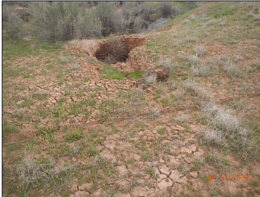
Hole and evidence of erosion moving soil and storm water off the SE side edge of location
