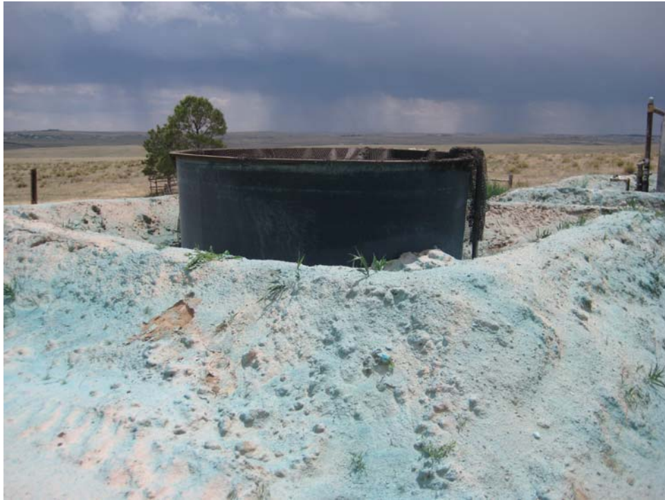
Photo 3. Fiberglass tank and berm
