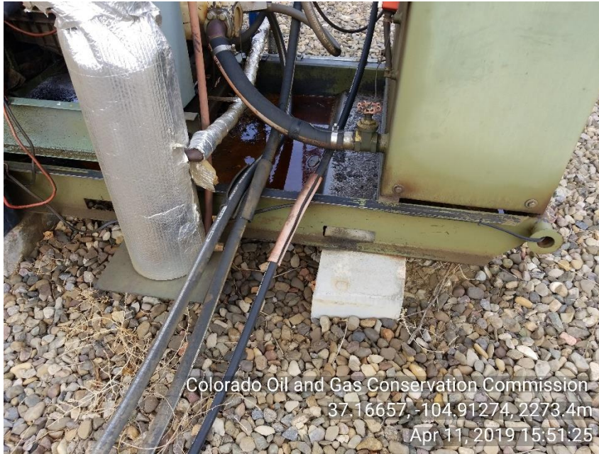
Photo 3 stained soil around HYD motor skid
