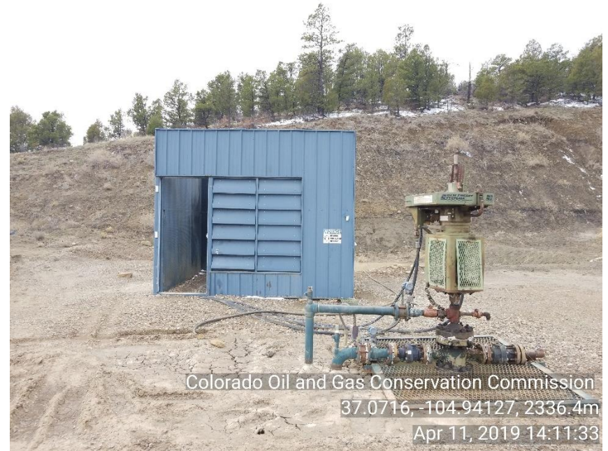
Photo 2 WH and HYD skid sound walls
