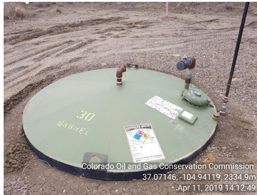
Photo 4 30bbl production tank with bull plug on load line
