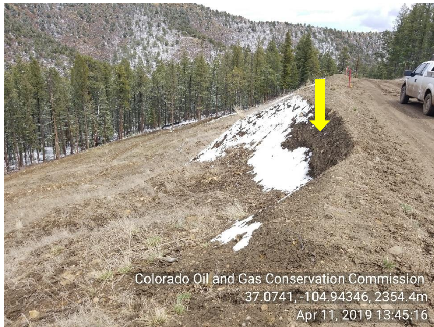
Photo 5 Storm water; location is eroding down hill side.
