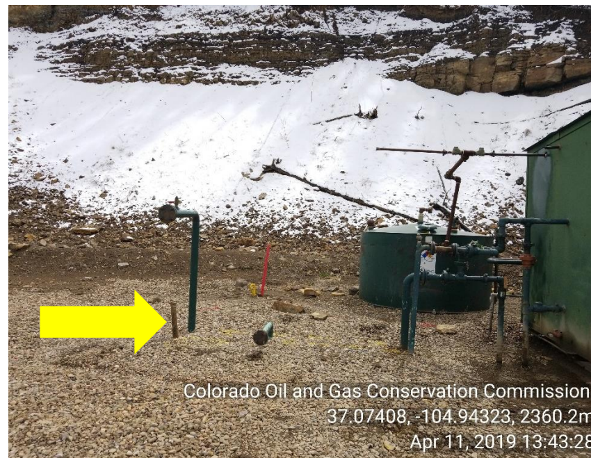
Photo 2 Unused, unmarked not LOTO risers
