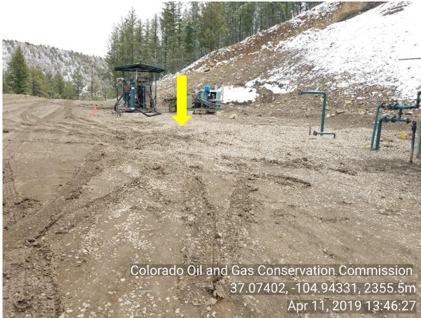
Photo 7 Storm water; Appears ditch line is settling deep ruts
