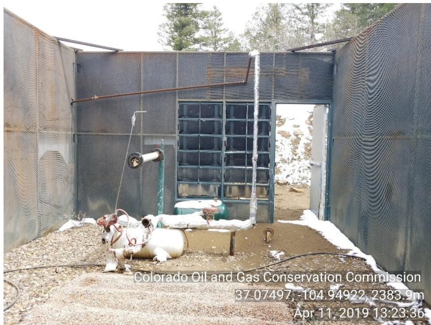
Photo 3 Unmarked, unused and not LOTO risers
