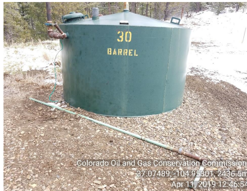
Photo 2 30bbl Produced water tank. Unused equipment 1' pipe
