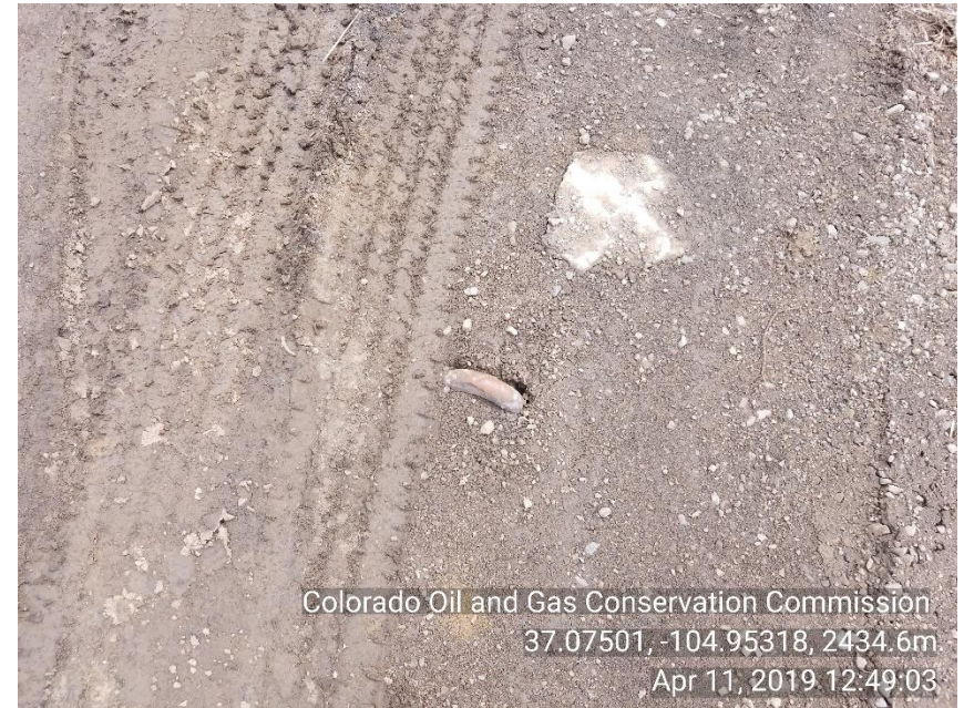
Photo 6 guy line anchor not properly marked.
