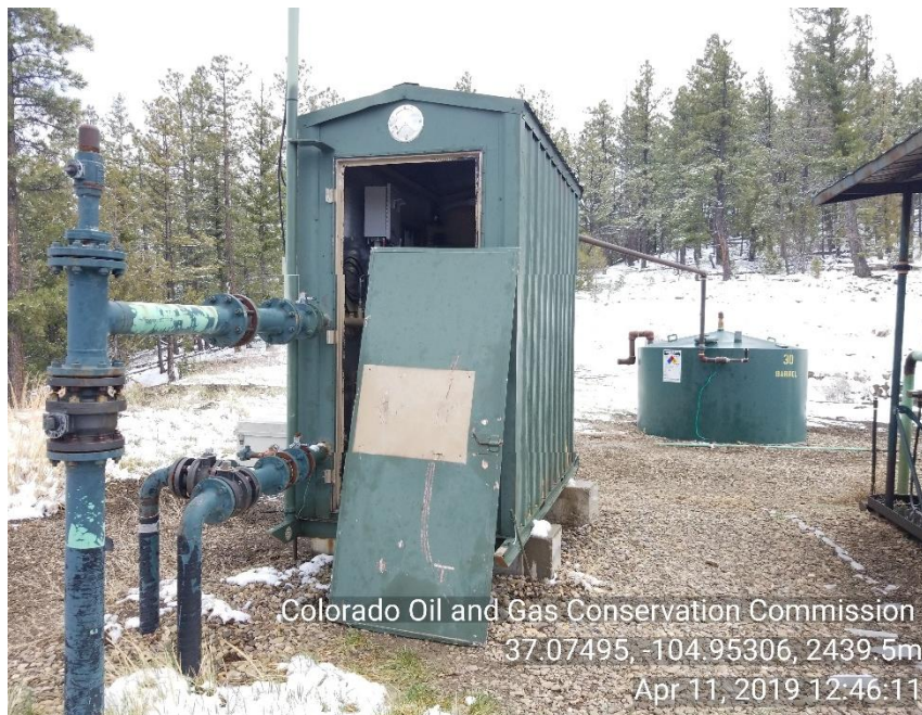
Photo 1 Sep/meter house. No well sign. Trash (door)
