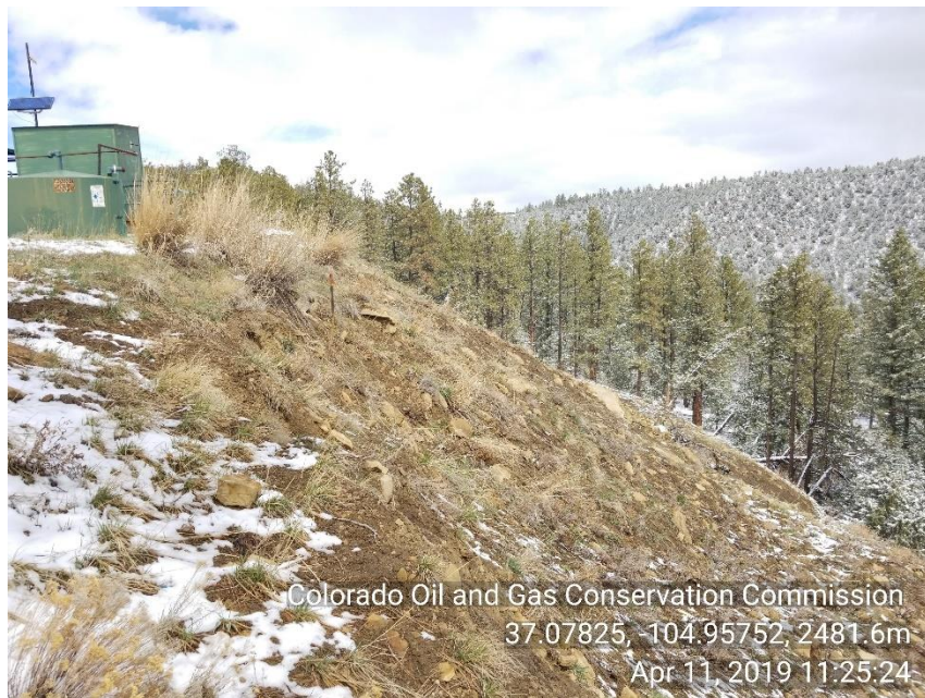
Photo 9 South east corner fill side of location appears to have broken away from location and slid down hill side.
