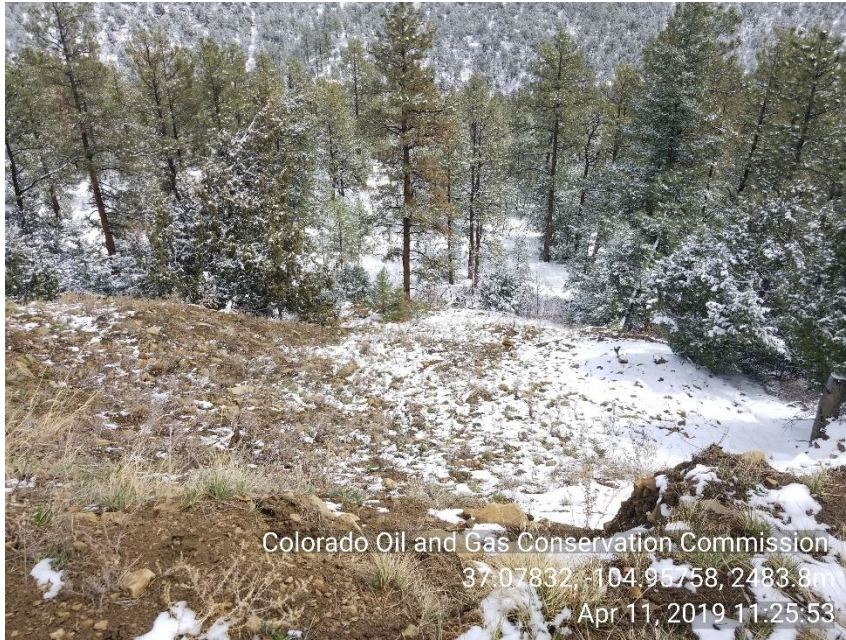
Photo 11 South east corner fill side of location appears to have broken away from location and slid down hill side.
