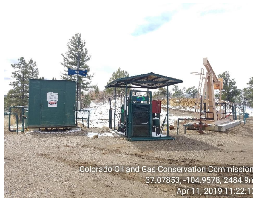
Photo 2 loc pic. Rods appear to have been removed from well. Pump jack not being used.
