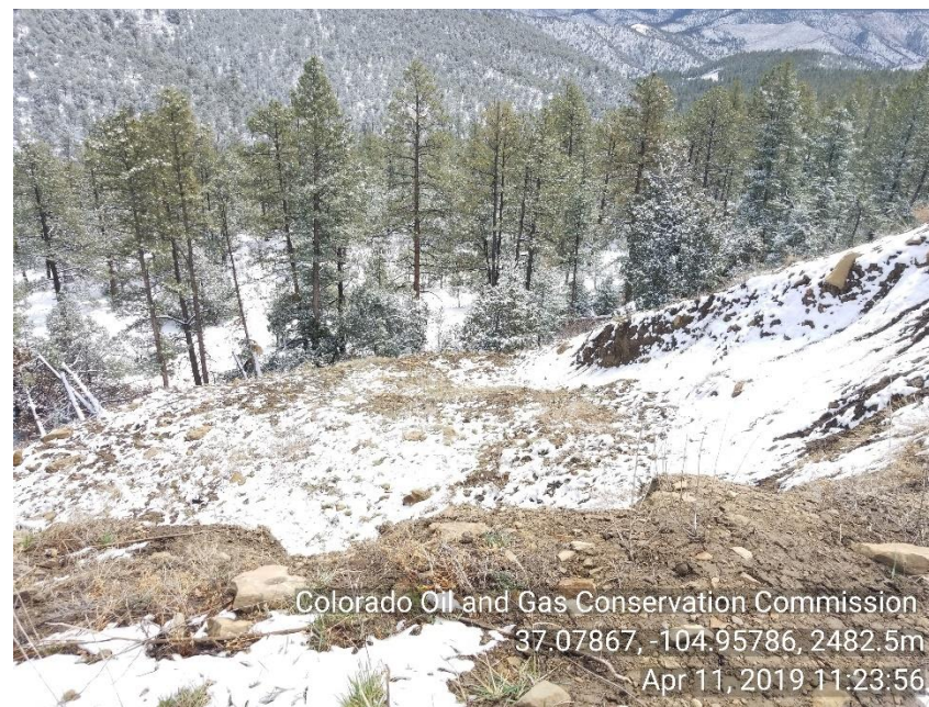
Photo 6 North east corner fill side of location appears to have broken away from location and slid down hill side
