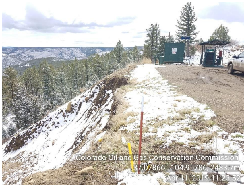
Photo 5 North east corner fill side of location appears to have broken away from location and slid down hill side.
