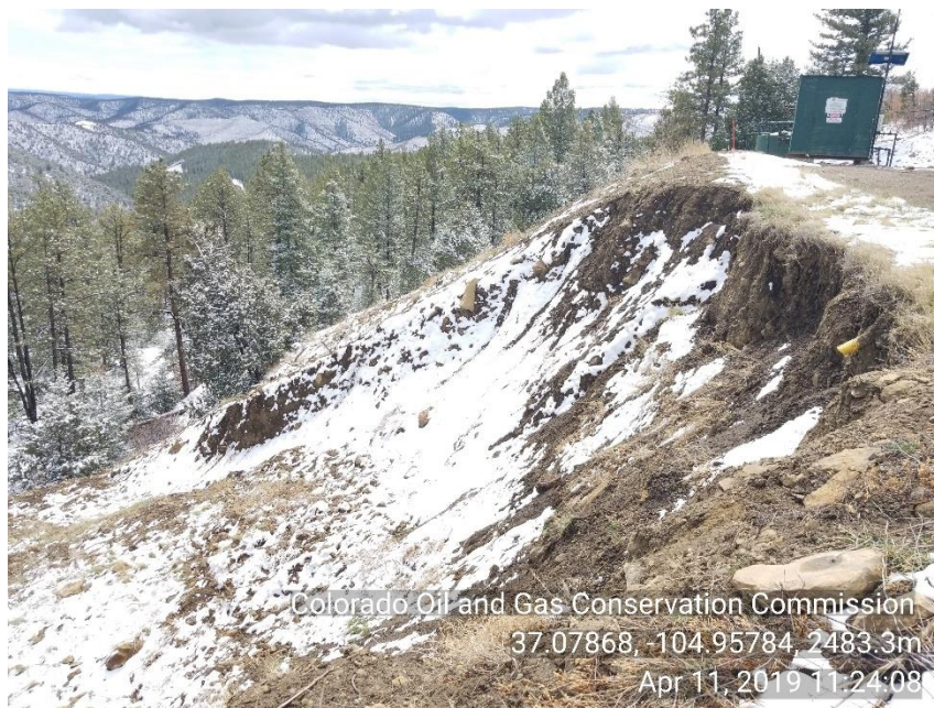
Photo 7 North east corner fill side of location appears to have broken away from location and slid down hill side.
