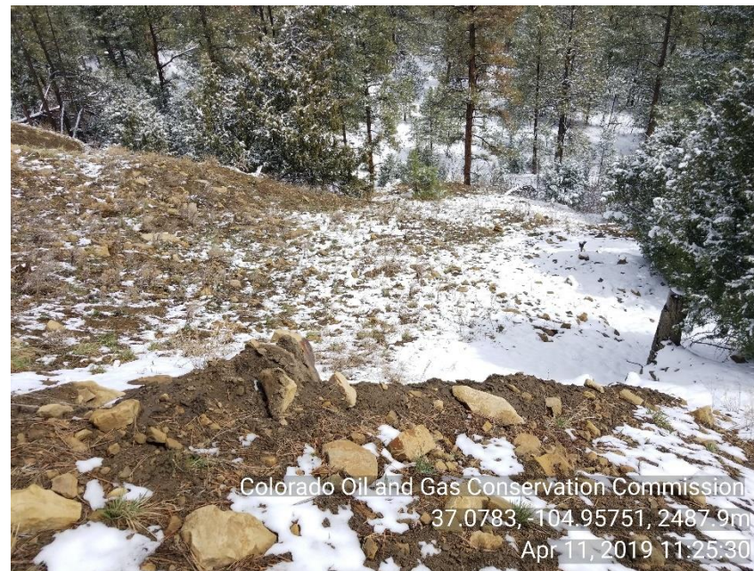
Photo 10 South east corner fill side of location appears to have broken away from location and slid down hill side.
