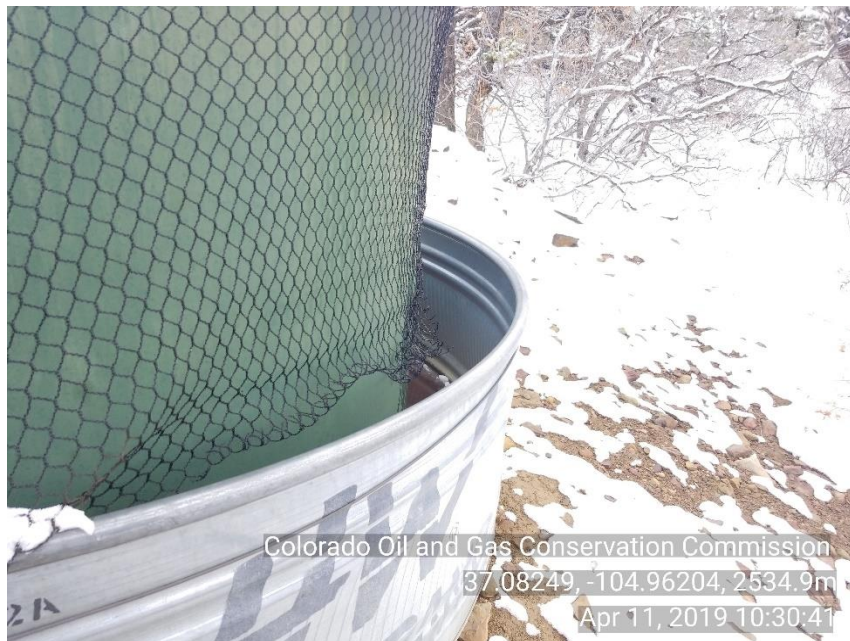
Photo 3 Bird netting on 20bbl tank secondary containment in disrepair.
