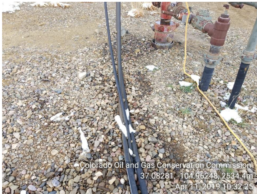
Photo 5 Stained soil around WH it appears from HYD lines
