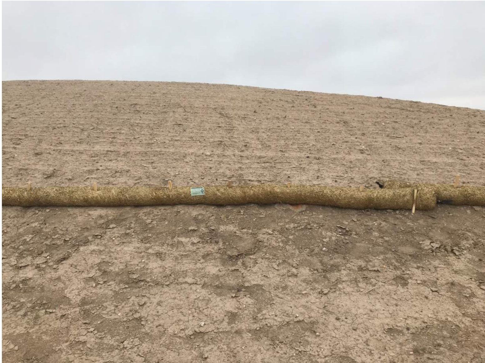
Erosion riling corrected and additional BMPs installed to topsoil stockpile. Looking east at topsoil pile.
