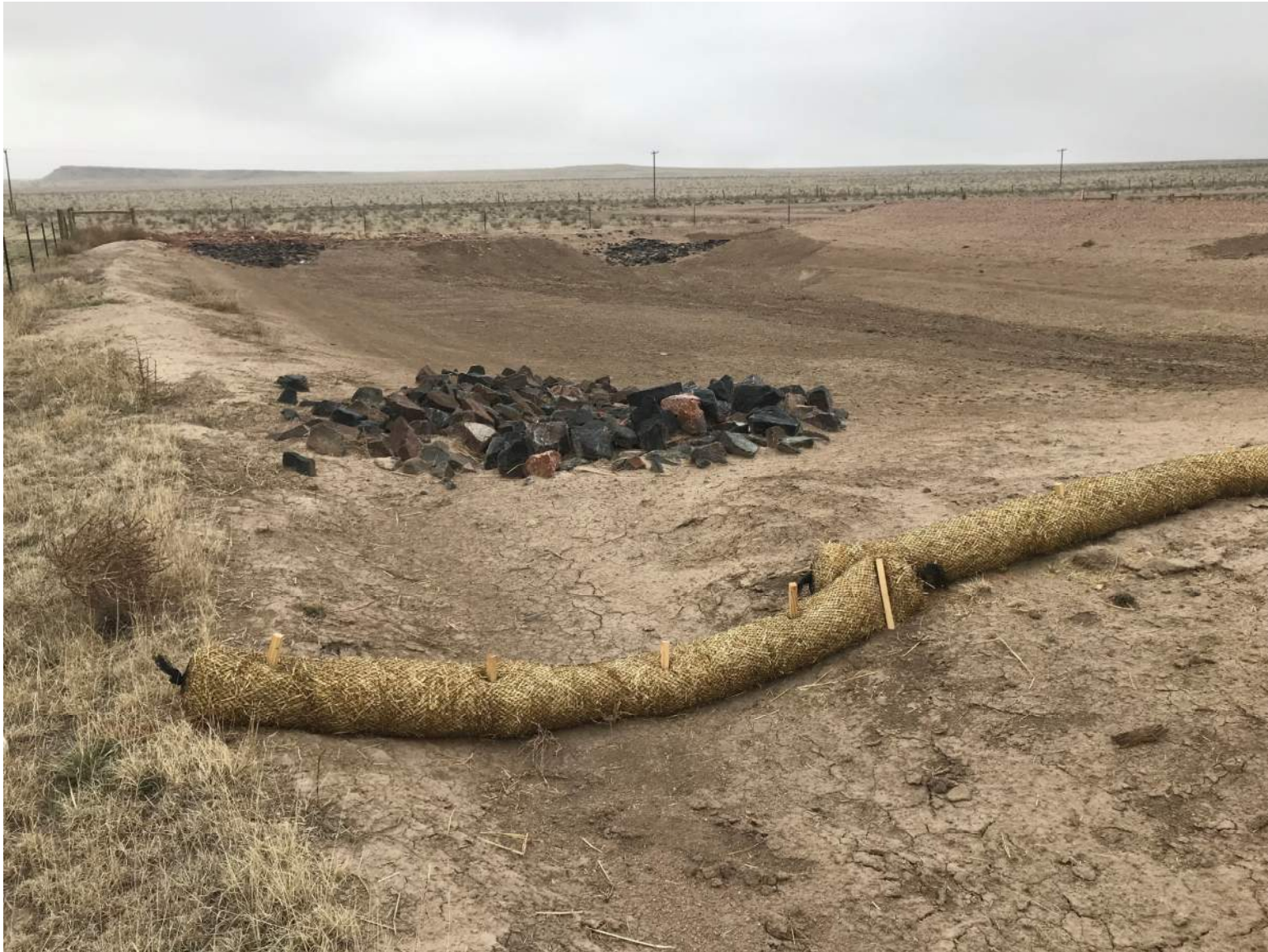
Sediment trapped cleaned, additional BMPs installed. Standing at the northeast corner of the sediment trap looking south.
