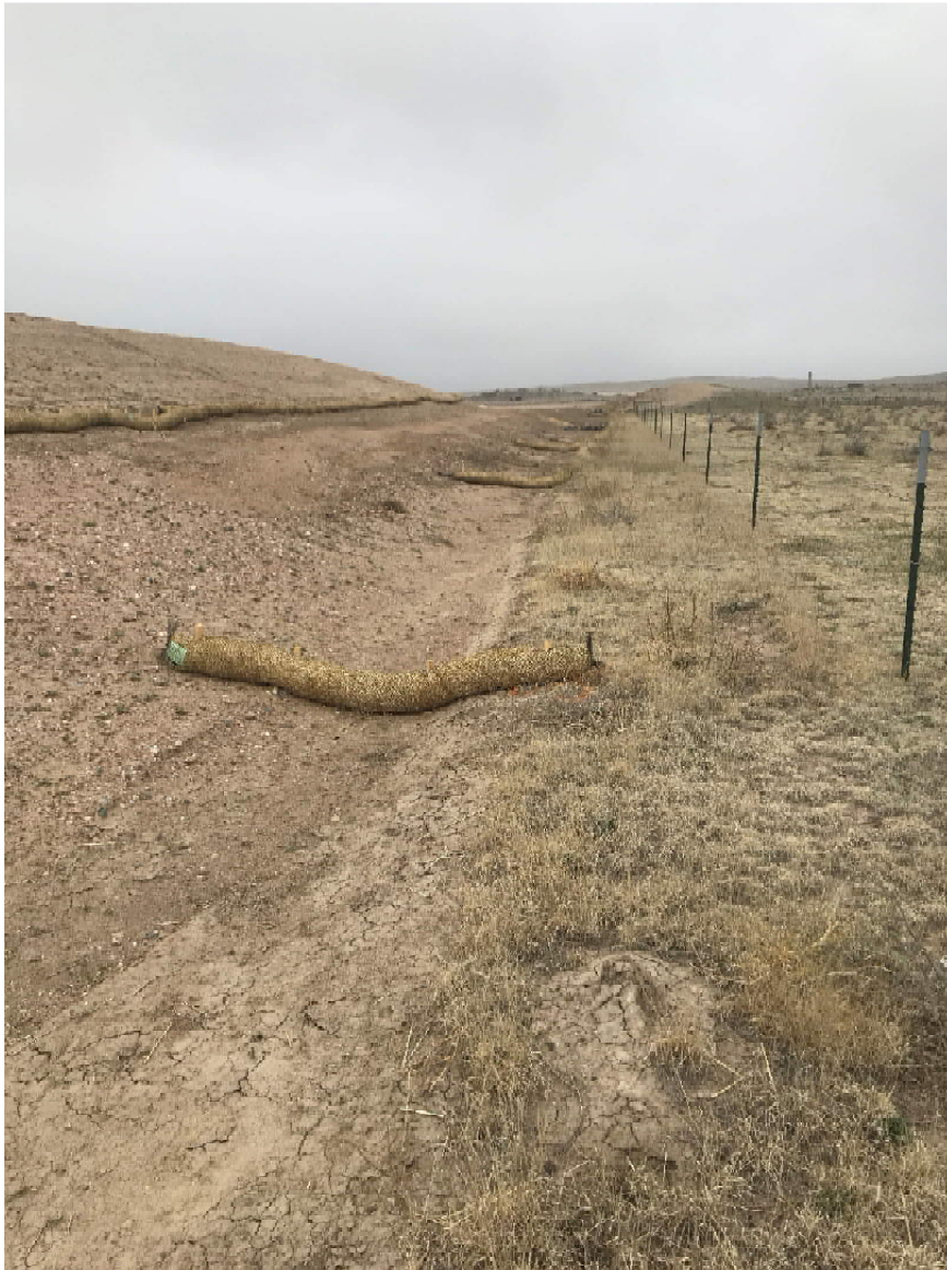
East perimeter ditch cleaned and additional BMPs installed. Looking north.
