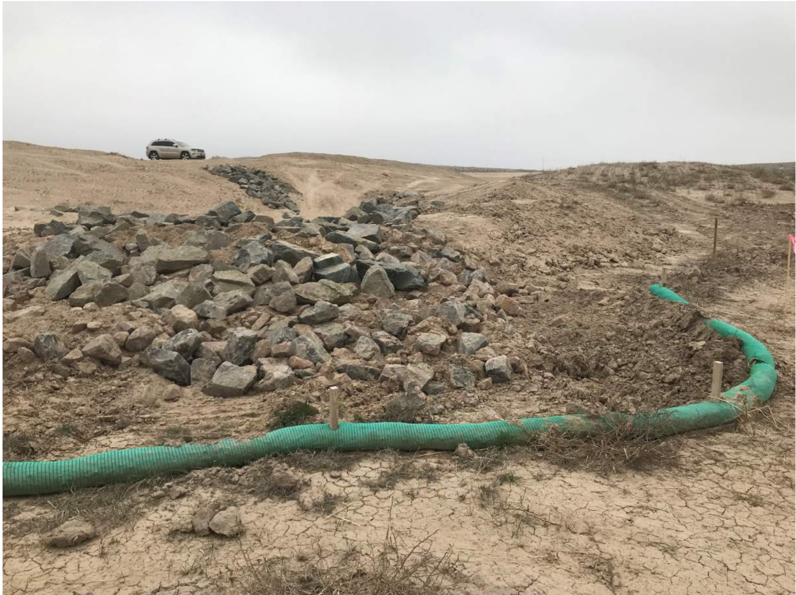
Standing in the south corner of the location, looking north at the sediment trap outlet. Can see the riprap rundowns from top of pad into sediment trap.
