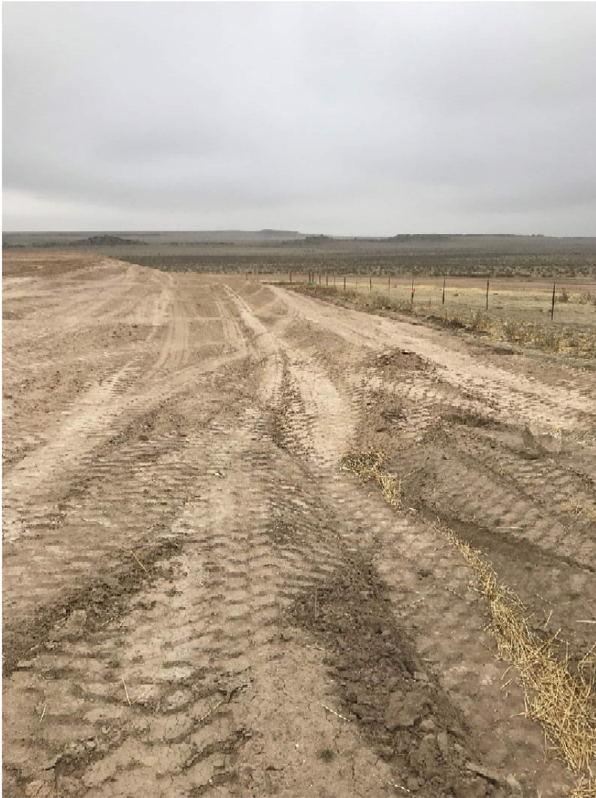
Start of capture swale mid fill slope. Standing near entrance looking southwest.
