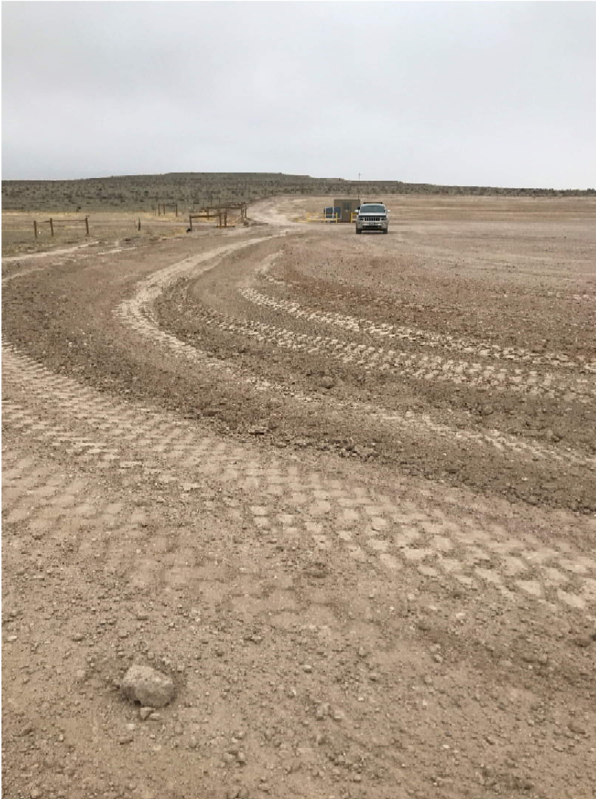
Cut ditch on top edge of pad. Standing at SE corner of pad looking towards entrance.
