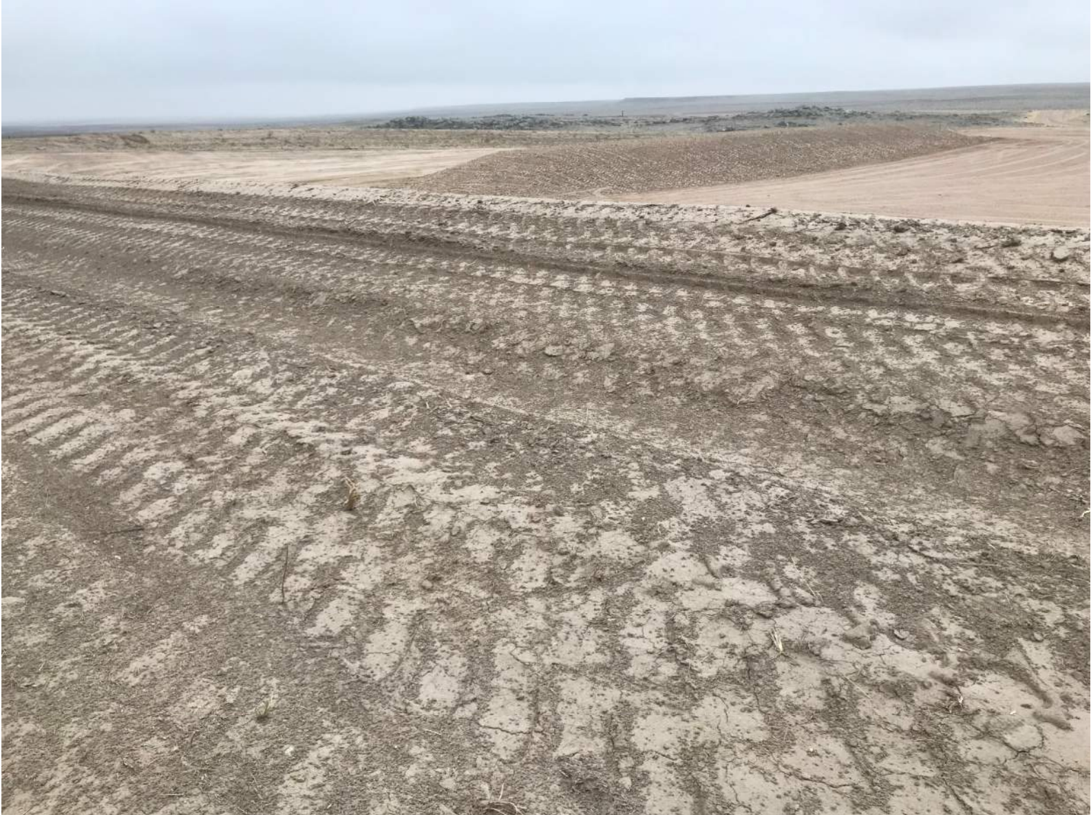
Ditch/berm on north edge of location at top of cut slope to re-direct run-on flows around the pad. Standing on north edge of location looking south.
