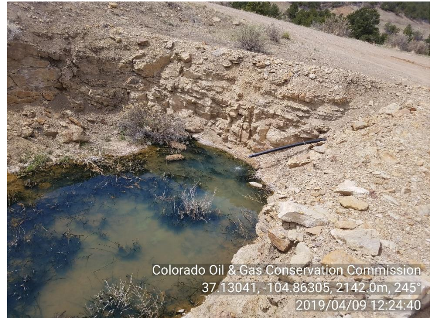
PHOTO 6: PHOTO SHOWING PIT LEVEL NOT FLUCTUATING DISPIE A SMALL STEADY STREAM OF PRODUCED CBM WATER FROM WELL BEING DISCHARGED INTO PIT.
