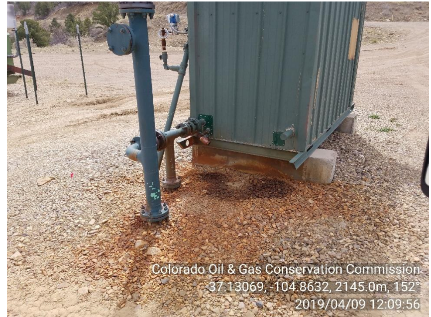
PHOTO 4: APPROXIMATELY 4' AREA OF IMPACTED SOIL ON NORTH SIDE OF METER HOUSE BENEATH SEPARATOR DRAIN. APPEARS BRODUCED CBM WATER IS BEING RELEASED FROM SEPARATOR.
