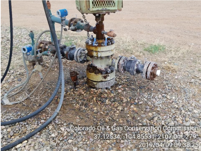
PHOTO 3: TBG PACKING IS LEAKING SPILLING PRODUCED WATER ON LOCATION NEAR WELLHEAD.
