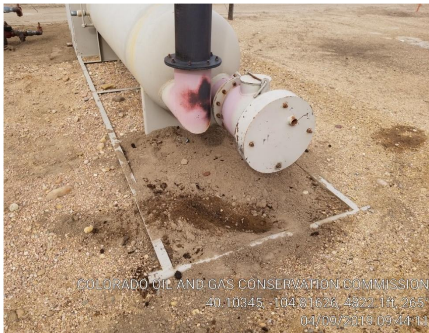
Pic 9 Appears to have stained soil under new soil.
