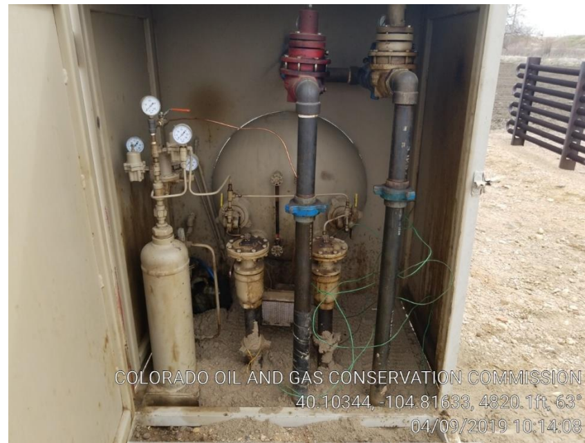
Pic 14 Inside of separator, leaking pipes appear to still be leaking. New soil appears to be covering stained soil.
