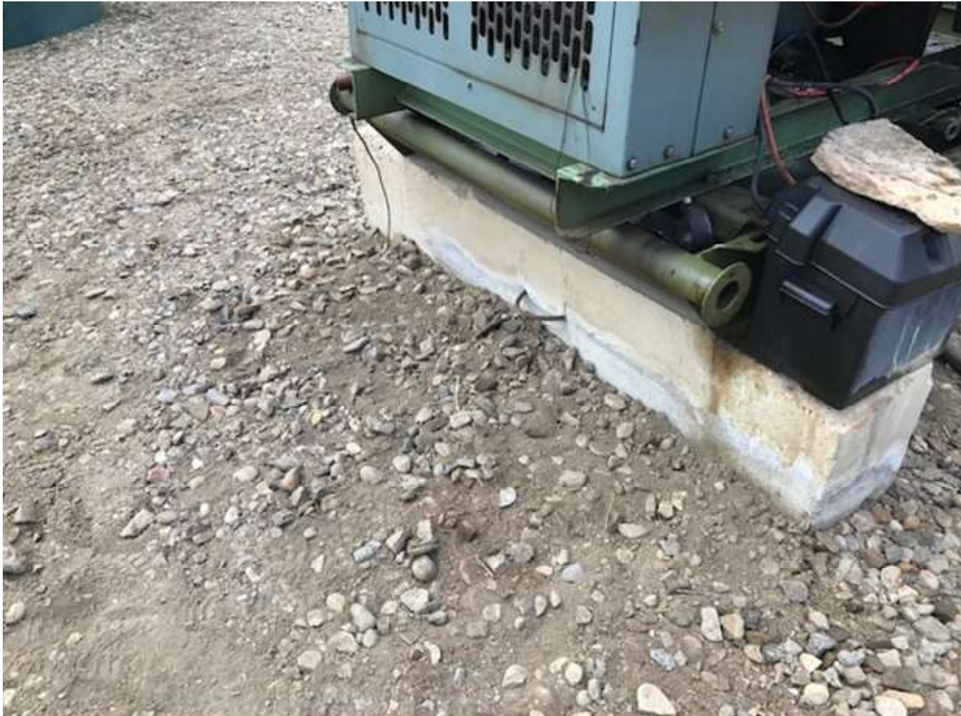
PHOTO 3: THE IMPACTED SOIL AROUND THE ENGINE SKID WAS REMOVED FROM LOCATION. ALL FITTINGS WERE SECURELY FASTENED TO ENSURE GOOD MECHANICAL CONDITION.
