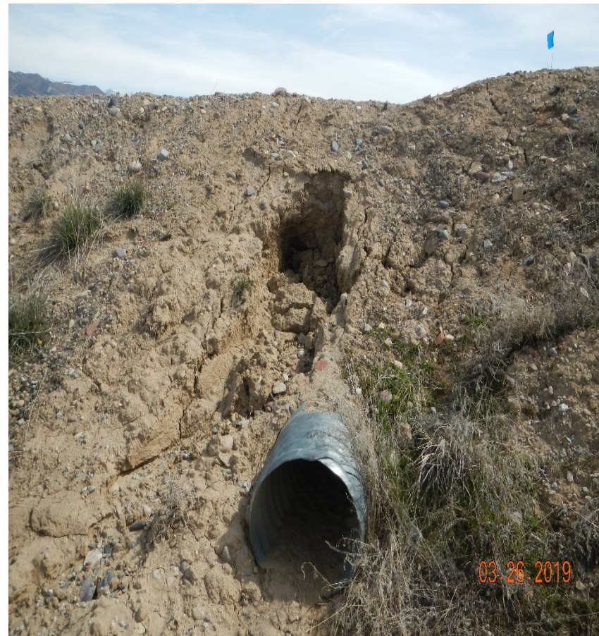
Photo#7: Ditch on West side of Access Road has failed
