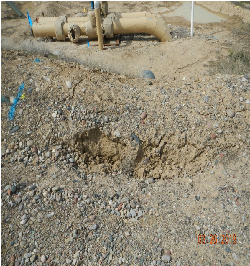
Photo#6: Ditch on West side of Access Road has failed
