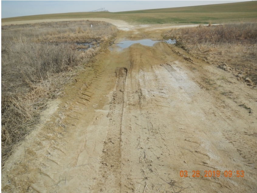
Photo 1. Photo taken from the access road, facing North. Appears the access road remains to the location and facility. Appears the culvert has failed and water is traversing the access road.
