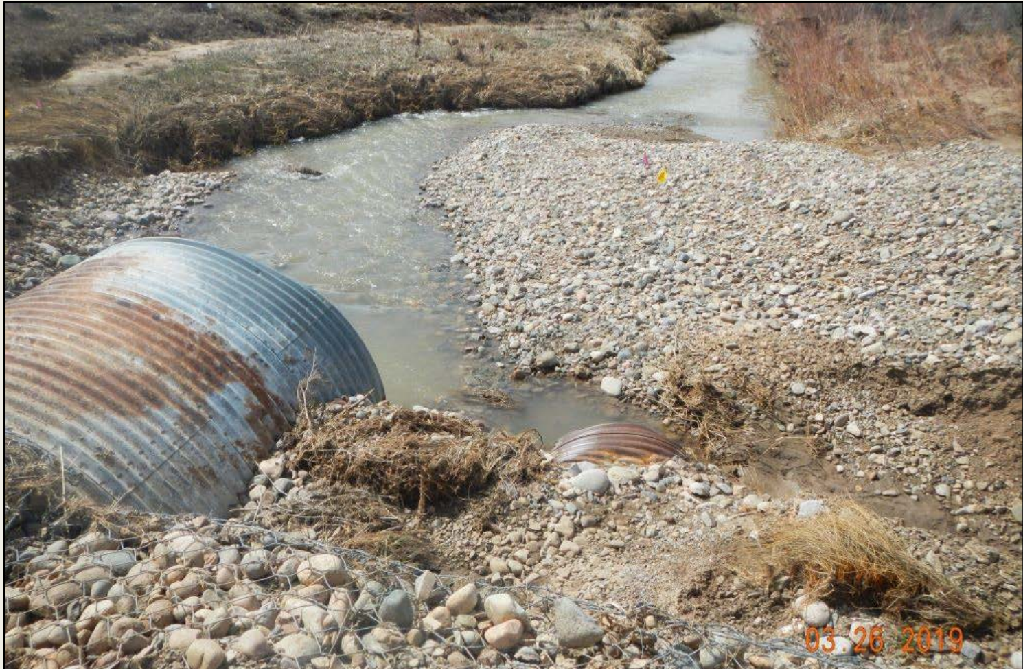
Photo 5. View of stream crossing where it appears significant sediment was recently discharged. Crossing is not stabilized, and culvert size is not adequate.
