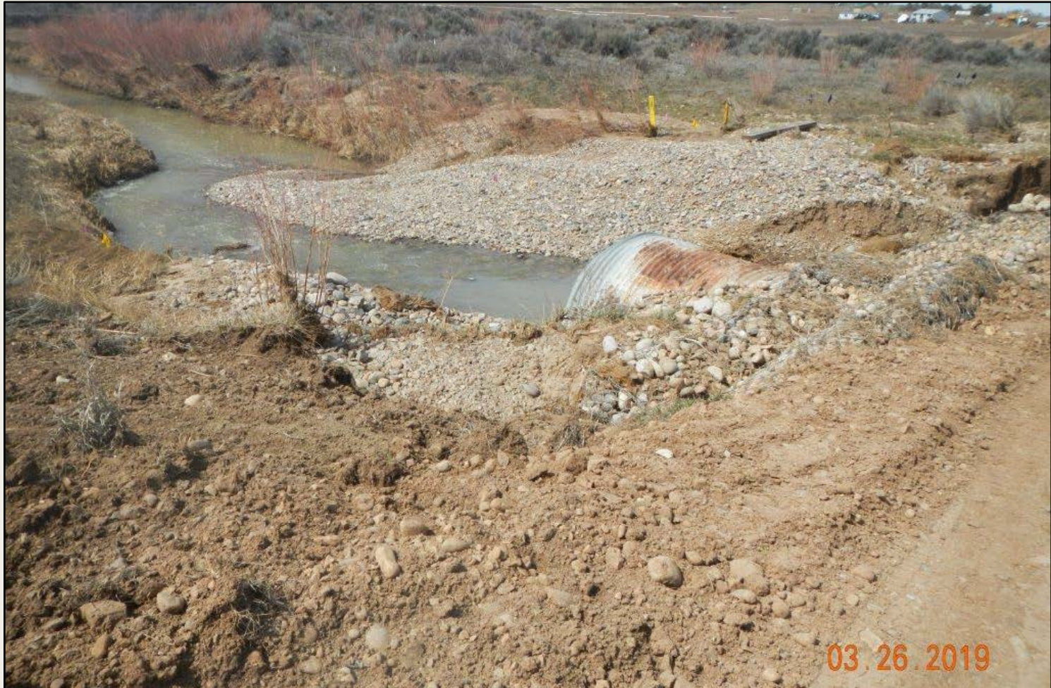
Photo 6. Another view of stream crossing showing loose soils and sediment/rock that appear to have recently been washed downstream.
