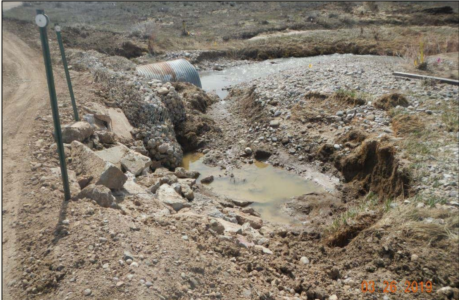
Photo 4. View of area along access at stream crossing that is eroding around culverts and is not stabilized. Culverts do not appear sufficiently sized to contain high flows and runoff events.
