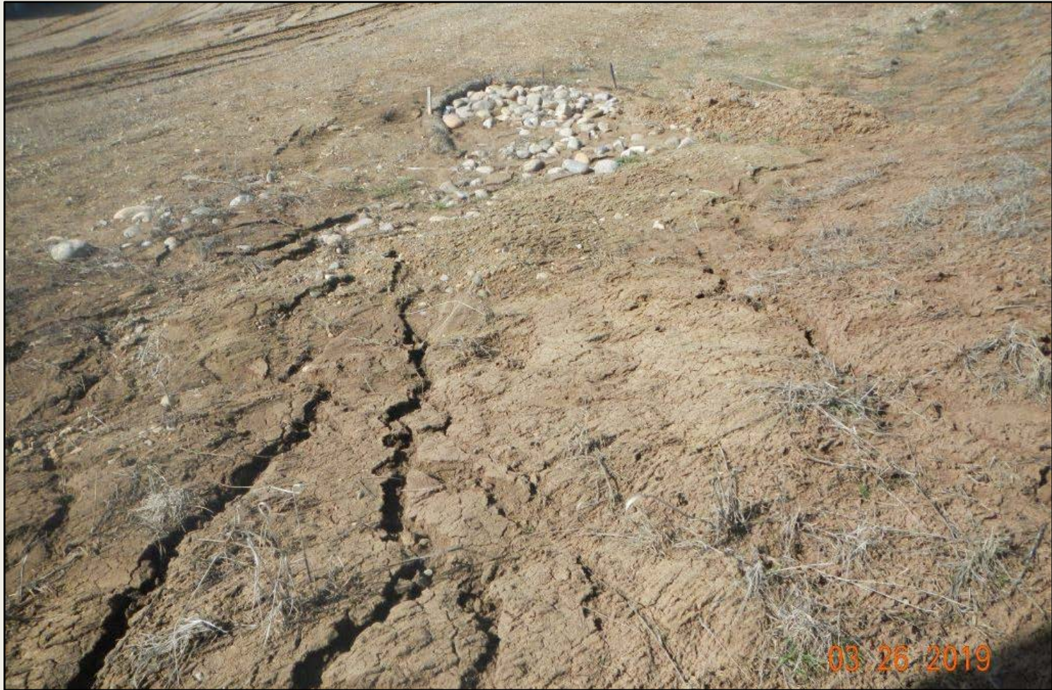
Photo 2. View of erosional rilling and sediment trap that are not functioning, north of the well pad entrance.
