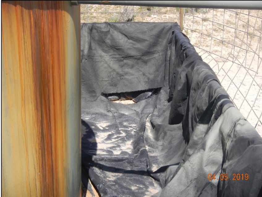
Photo #5 Pit liner with large rip or tear
