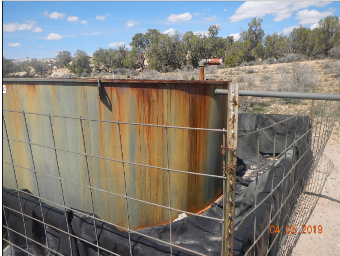
Photo #4 Tank needs paint and has a lot of rust.
