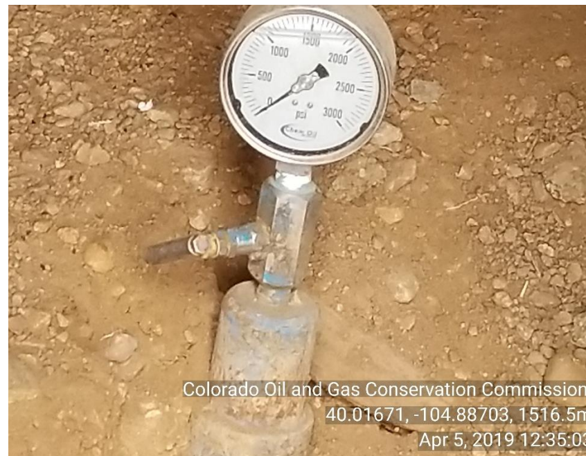
Photo 2 Braden head pressure 0psig
