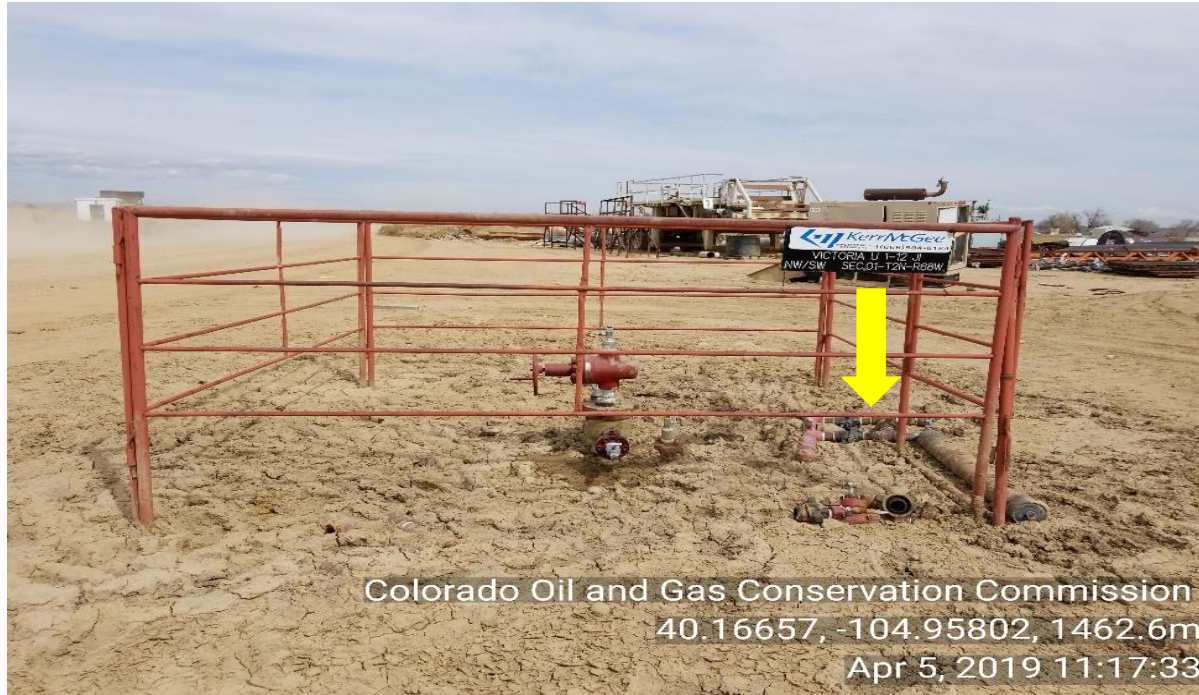
Photo 1 WH all production equipment has been removed. Unused equipment: plunger lift and piping
