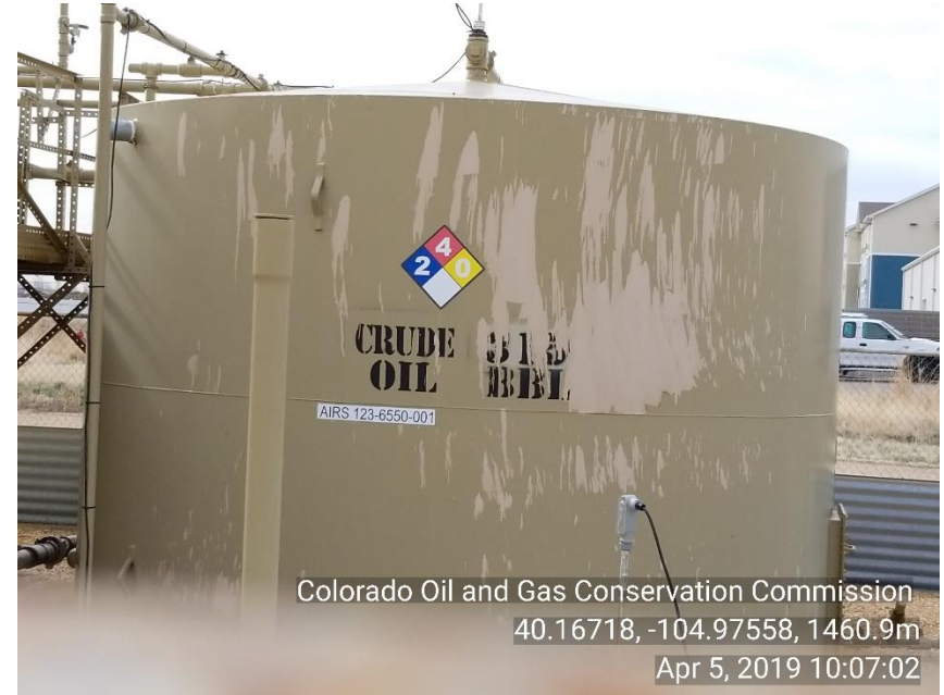
Photo 6 Volume label not legible. Visual impact paint is in disrepair. Tank visible from I-25 and in close proximity to office buildings.
