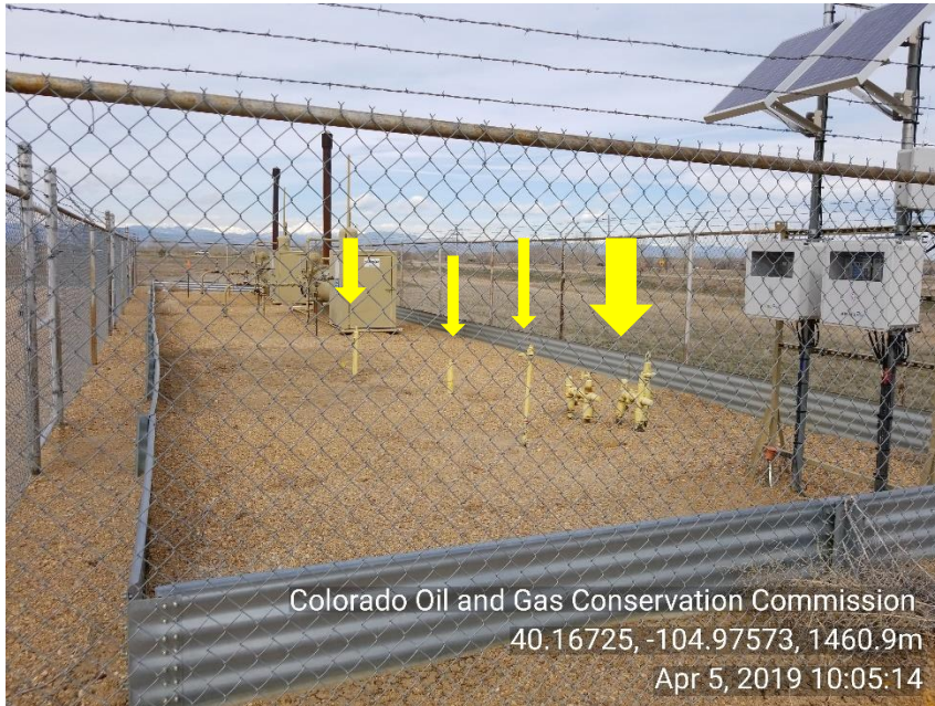
Photo 3 Separators and unmarked, unused and not LOTO risers.
