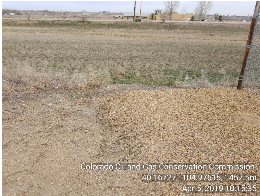
Photo 11 Storm water reels on North west side of location carrying sediment off location
