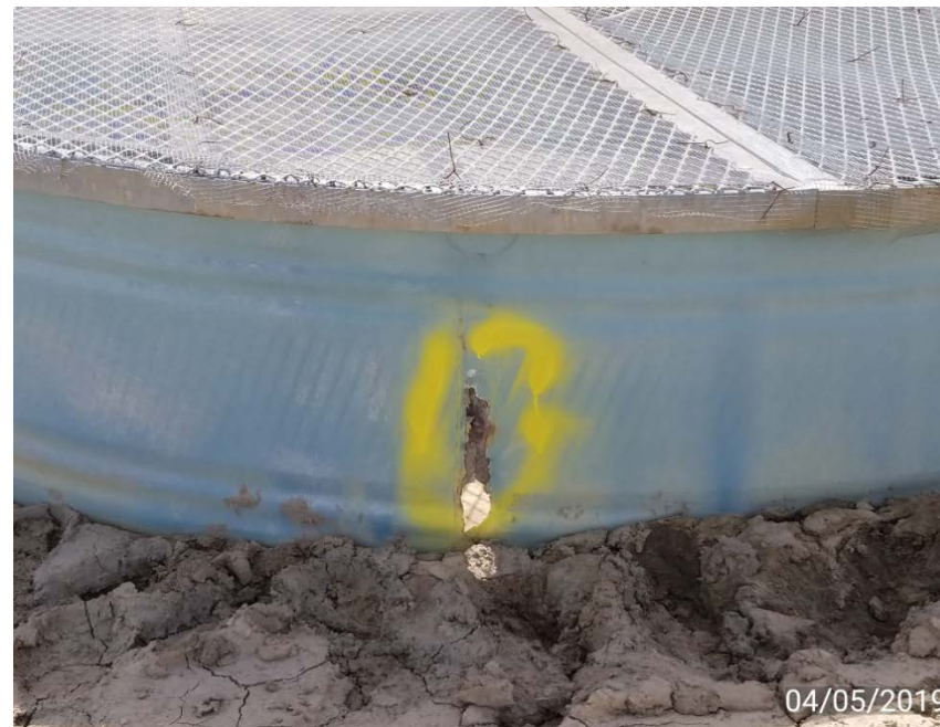
Photo 2. Hole in tank.
