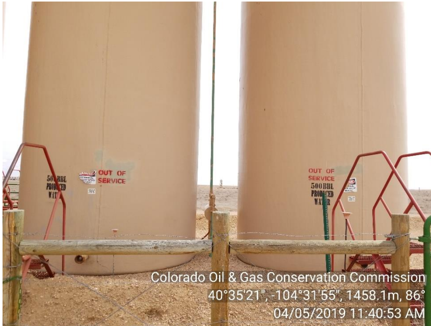
Photo 3: No placarding on produced water tanks
