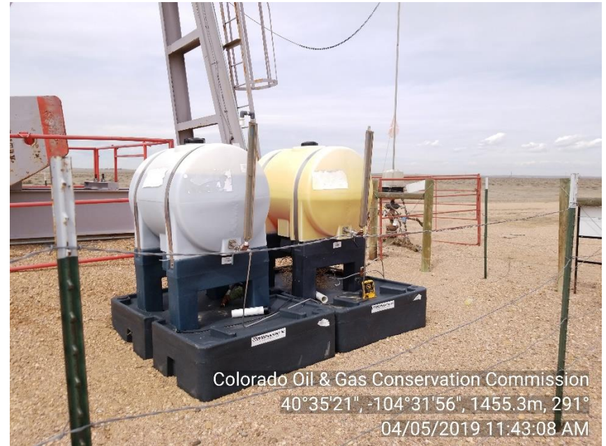
Photo 4: No labeling on chemical barrels.
