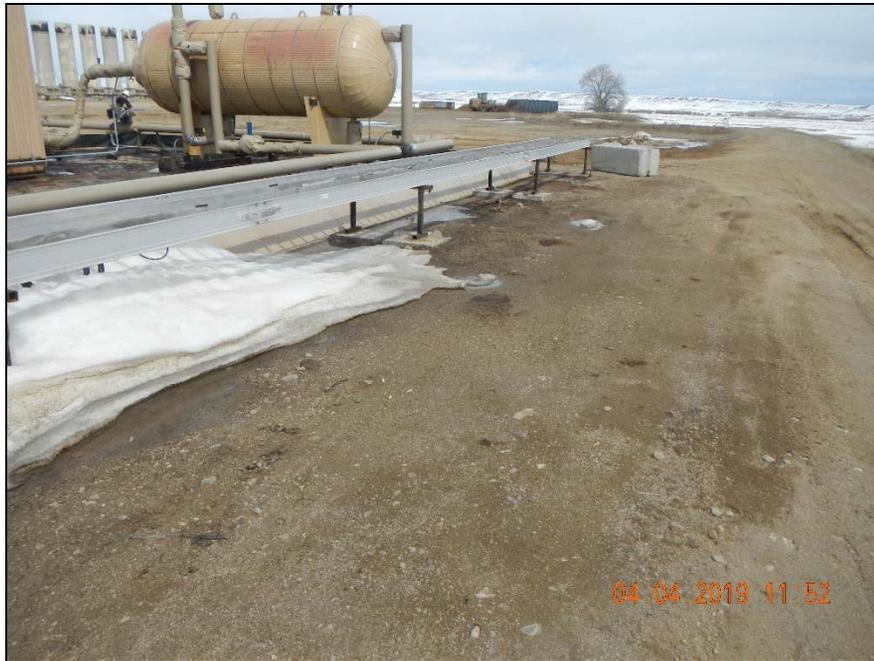
**Photo 19. Non-reportable spill, stained soil outside containment.**
