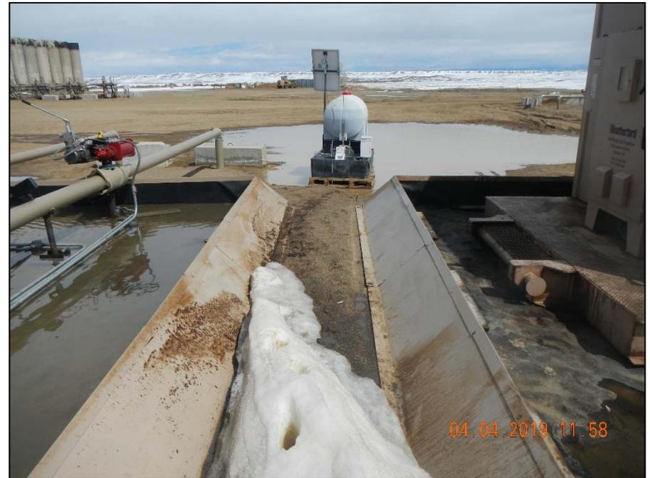
**Photo 22. Non-reportable spill, stained soil outside containment. Containment on left contains snowmelt, containment on right does not.**
