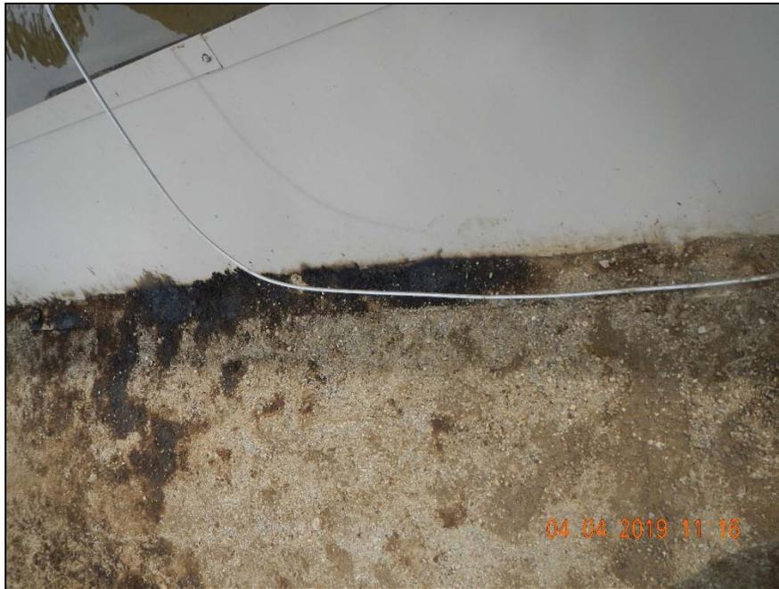
**Photo 17. Non-reportable spill, stained soil outside containment.**
