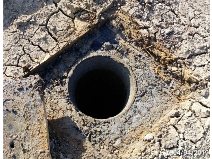
Photo 4. Well casing without cover.
