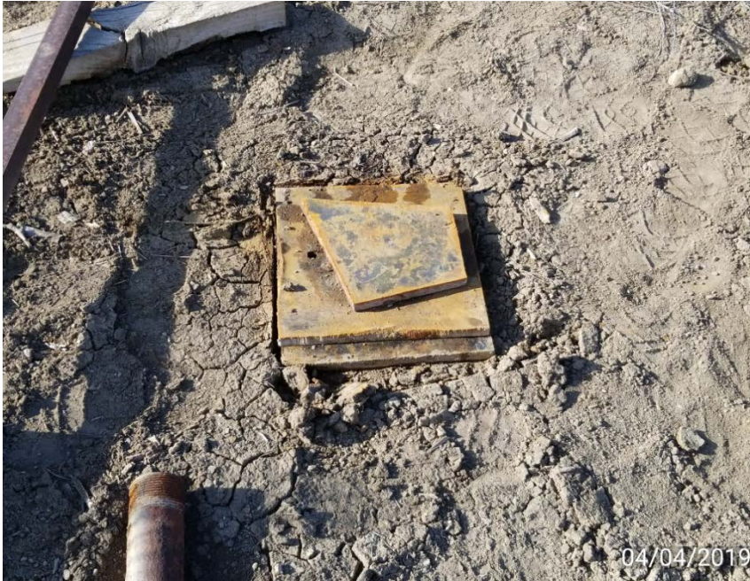
Photo 3. Well casing covered with steel plate.
