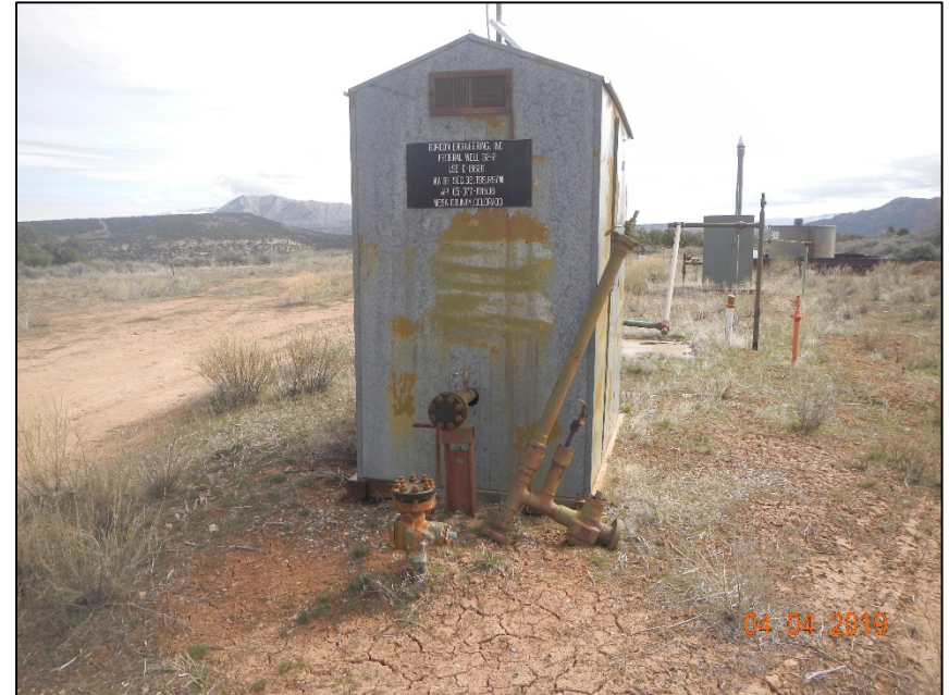
Photo #9. Unused equipment. Gas Meter appears to be disconnected. Risers are not marked or locked out tagged out.
