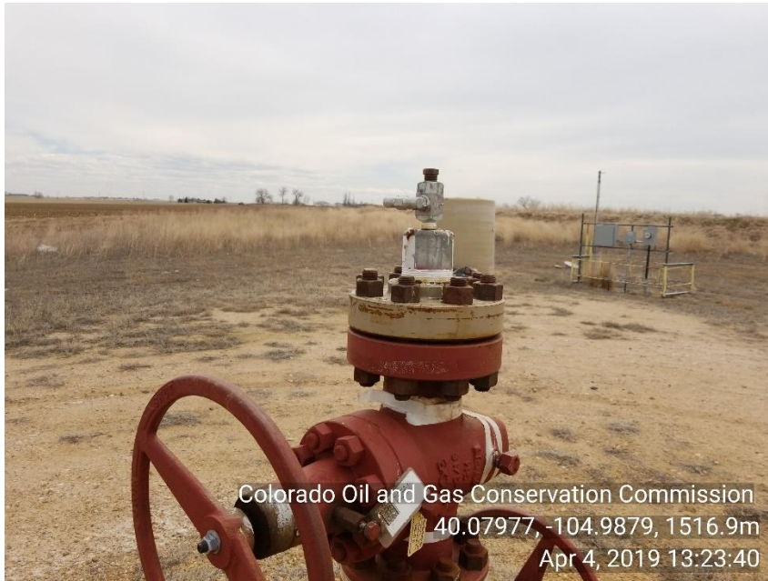
Photo 3 no gauge on top of WH
