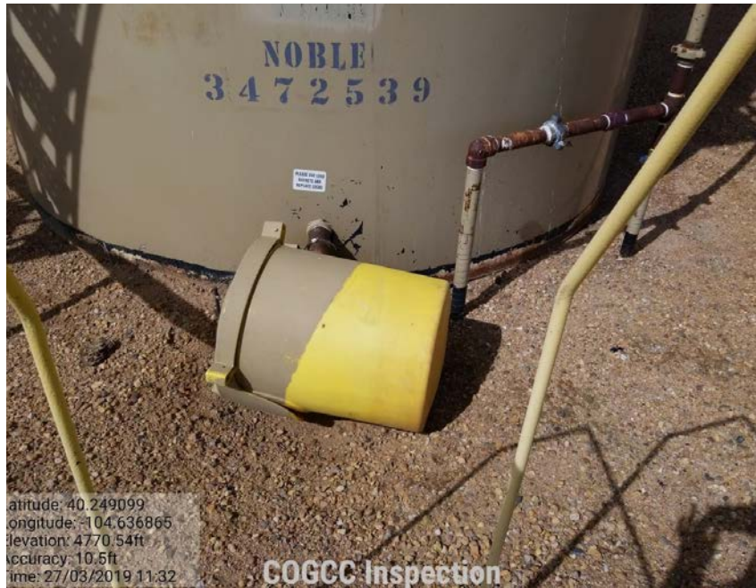
Photo 7 – Drip pan on crude tank load out damaged.
