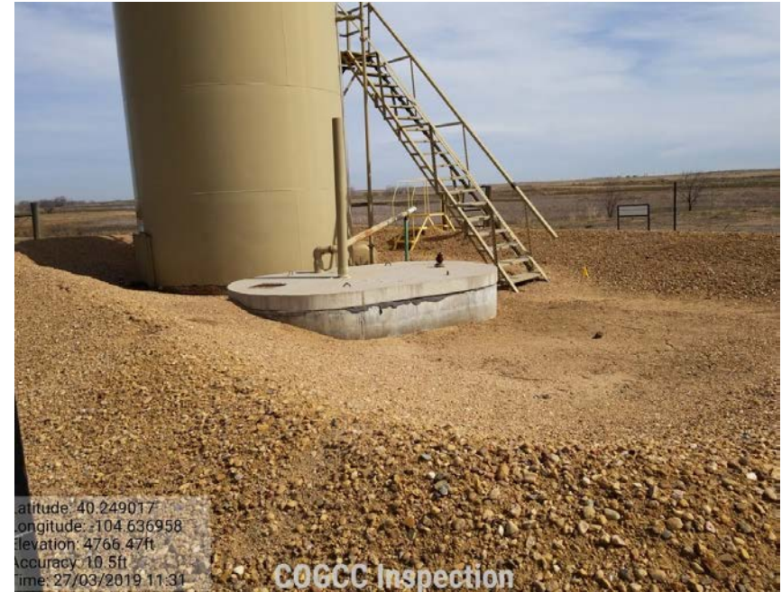
Photo 6 – Produced water vault and crude storage tank within secondary containment.
