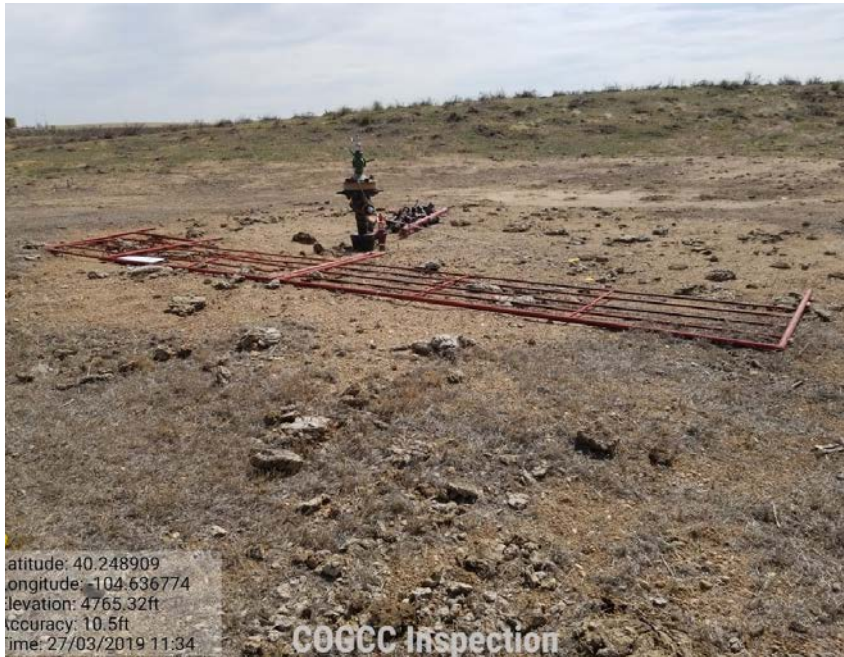
Photo 3 – Jepsen 3 wellhead (123-13646). Fencing and signage down. Well marked as long term shut in. Form 6 on file indicating P&A on 11/03/2017 (Document #401473775).
