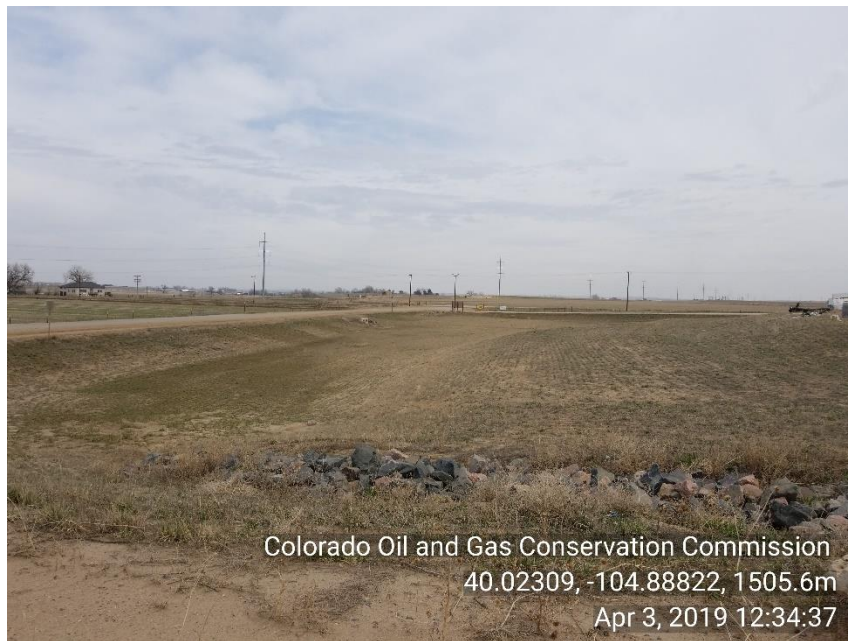
Photo 13 Drainage ditched rip raped and sediment trap
