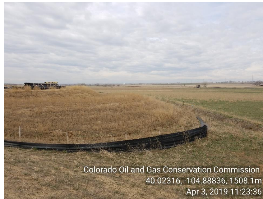
Photo 8 silt fence not maintained around perimeter of location
