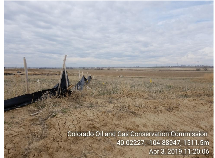
Photo 4 silt fence not maintained around perimeter of location
