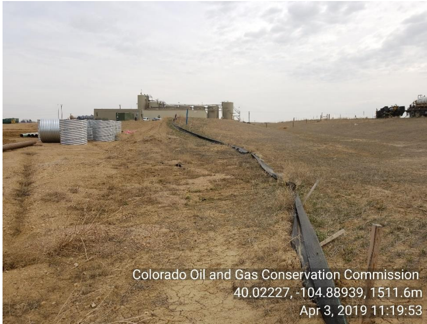
Photo 3 silt fence not maintained around perimeter of location
