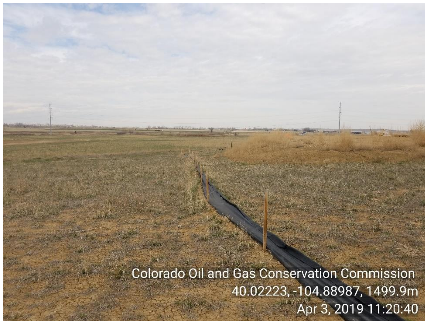
Photo 5 silt fence not maintained around perimeter of location
