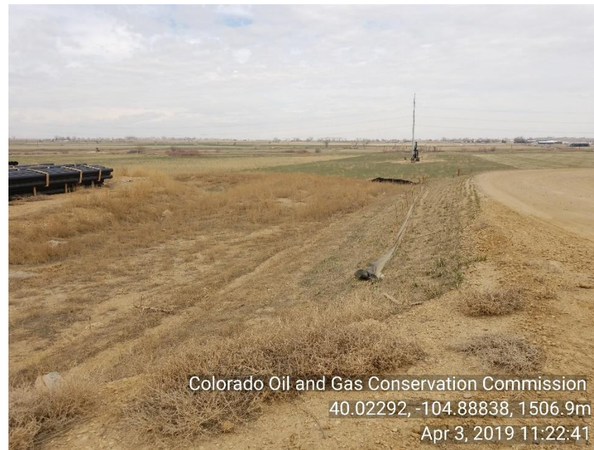
Photo 6 silt fence not maintained around perimeter of location
