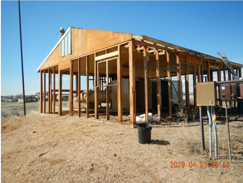
Photo 5: Production equipment building with siding and underlayment removed. The roof was in the process of being removed.
