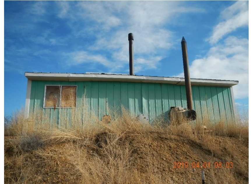
Photo 2: Production equipment building with separator heater stacks visible.
