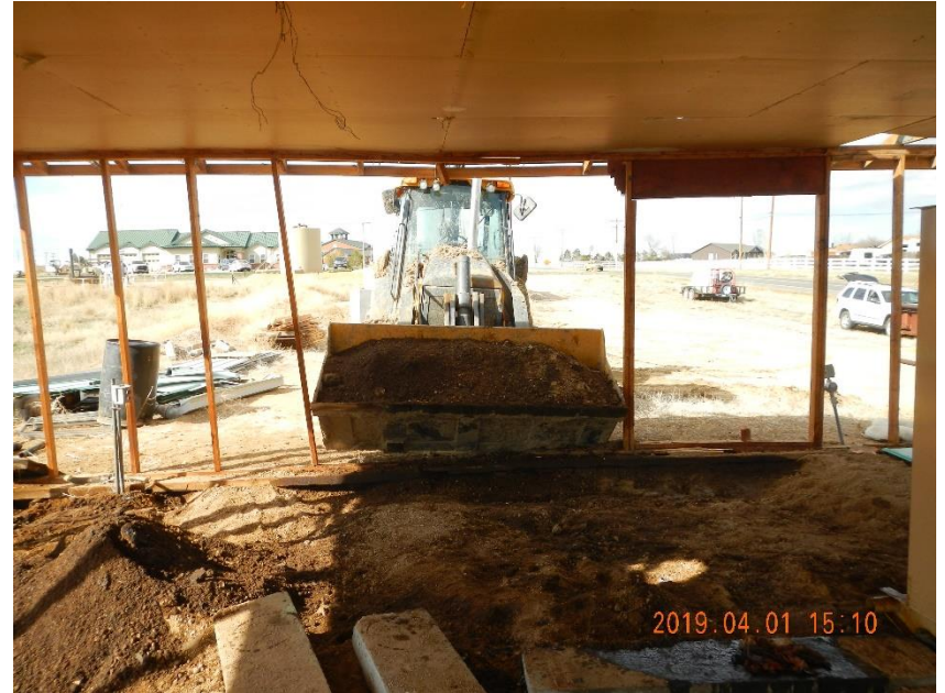
Photo 10: Removing impacted soil from release.
