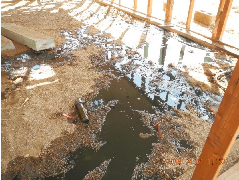
Photo 7: Fluid released from separator when valve broke off vessel.
