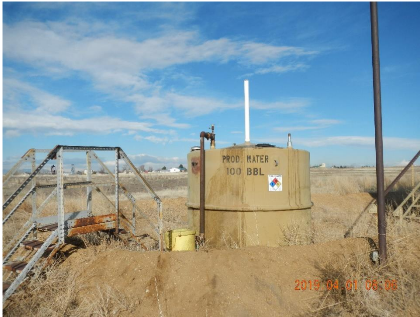
Photo 3: Produced water tank.
