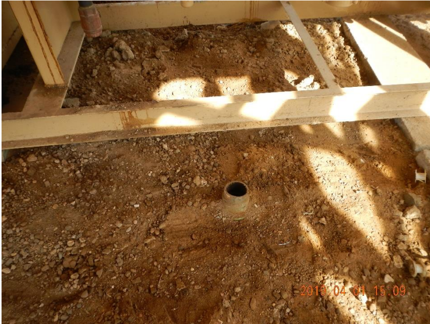
Photo 11: (1) of (2) open flow line/risers located inside building.
