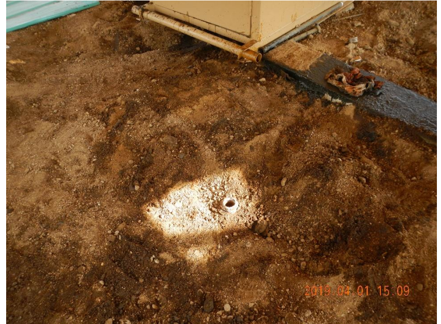
Photo 12: (2) of (2) open flow lines/risers located inside building.
