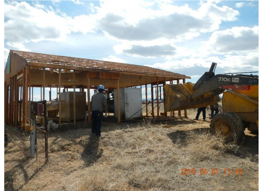
Photo 6: Pulling the W horizontal separator out of building.
