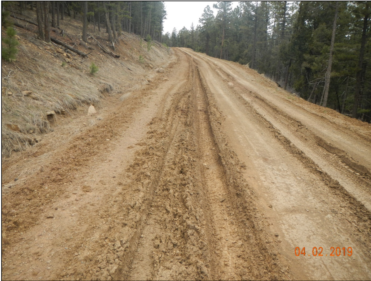
Photo 1. There is signs of erosion and vehicle rutting along the road that travels up to the location.
