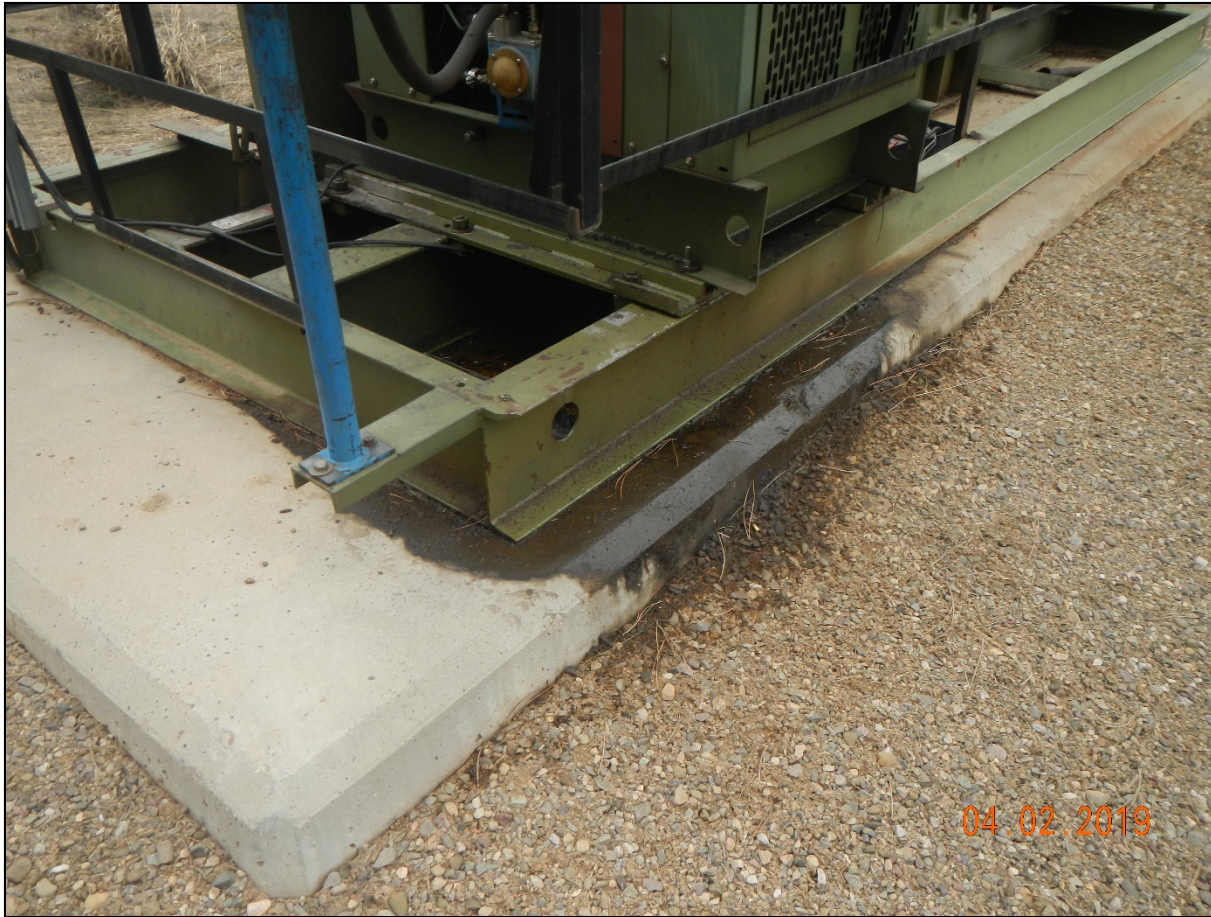
Photo 2. There is some oil on the engine skid.
