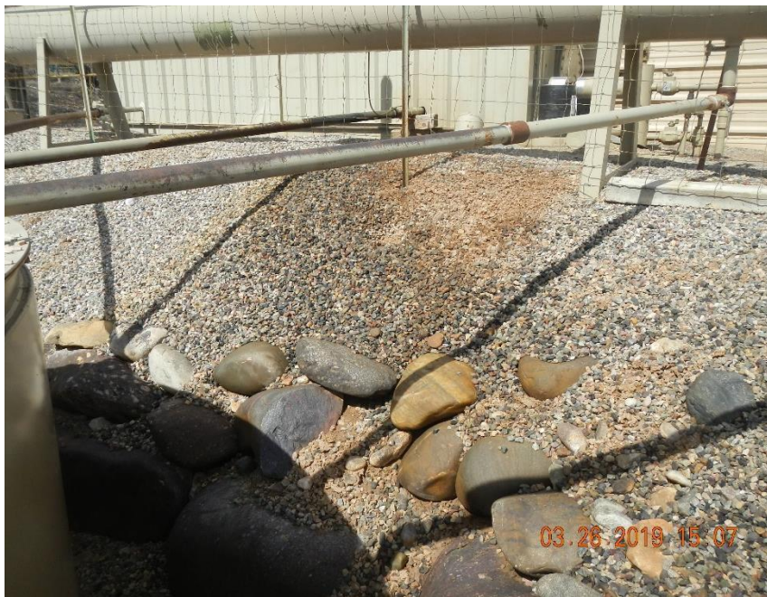
Stained gravel and rocks on north side of secondary containment area.
