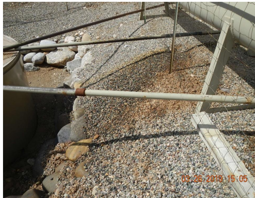
Stained soil north of open topped produced water tank.
