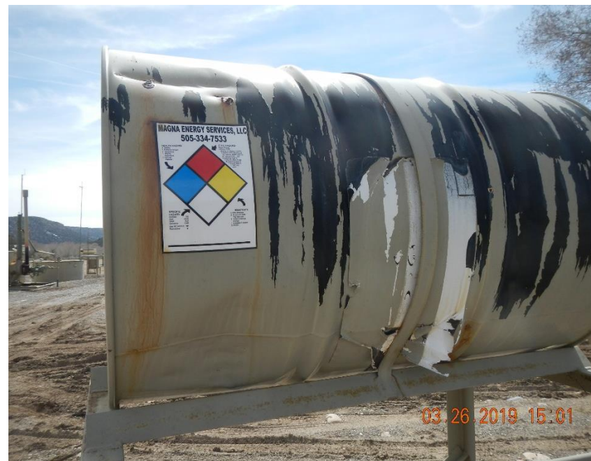
Unlabeled chemical container with blank NFPA placard.
