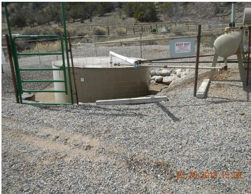
Open topped produced water vessel without required labeling.
