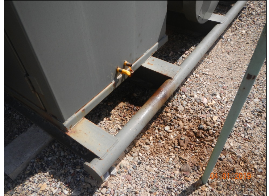
Stained soil around separators
