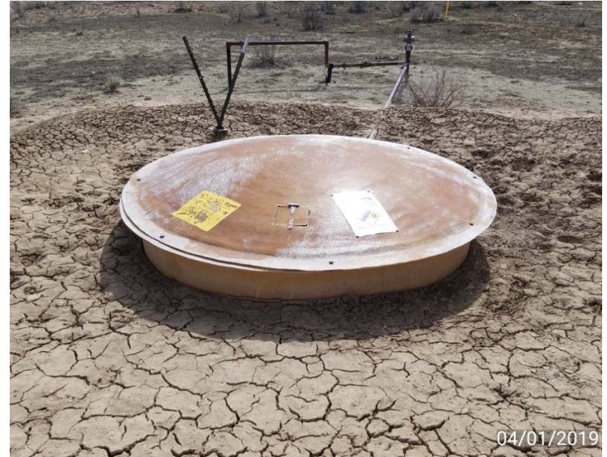
Photo 2. Blow down tank.
