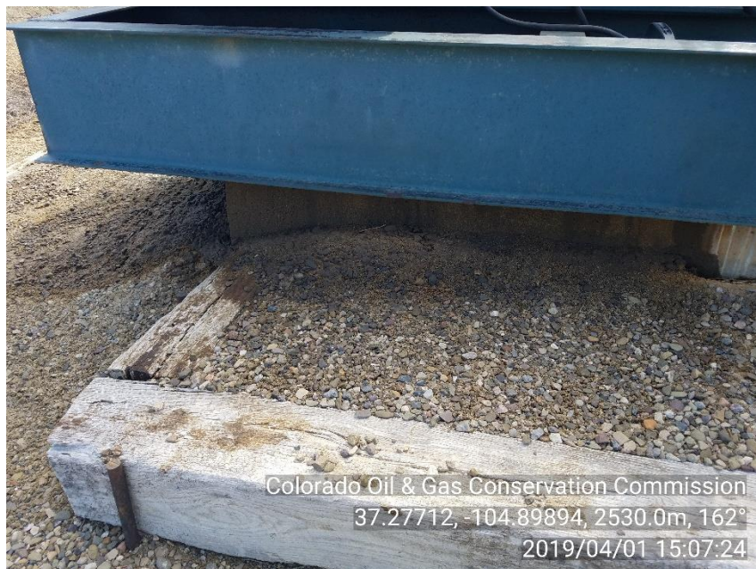
PHOTO 3: OIL IS LEAKING FROM PUMPJACK SKID AND CAUSING IMPACTED SOIL ALL AROUND PUMPJACK BASE
