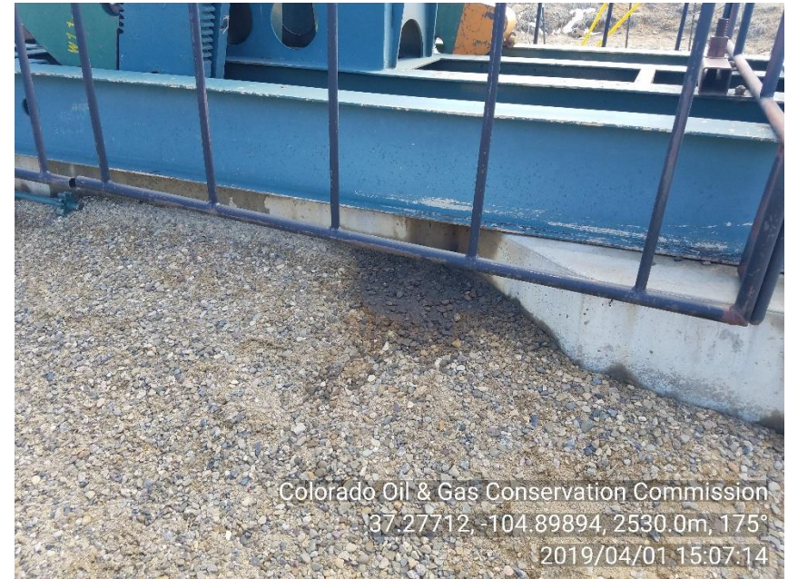
PHOTO 4: OIL IS LEAKING FROM PUMPJACK SKID AND CAUSING IMPACTED SOIL ALL AROUND PUMPJACK BASE
