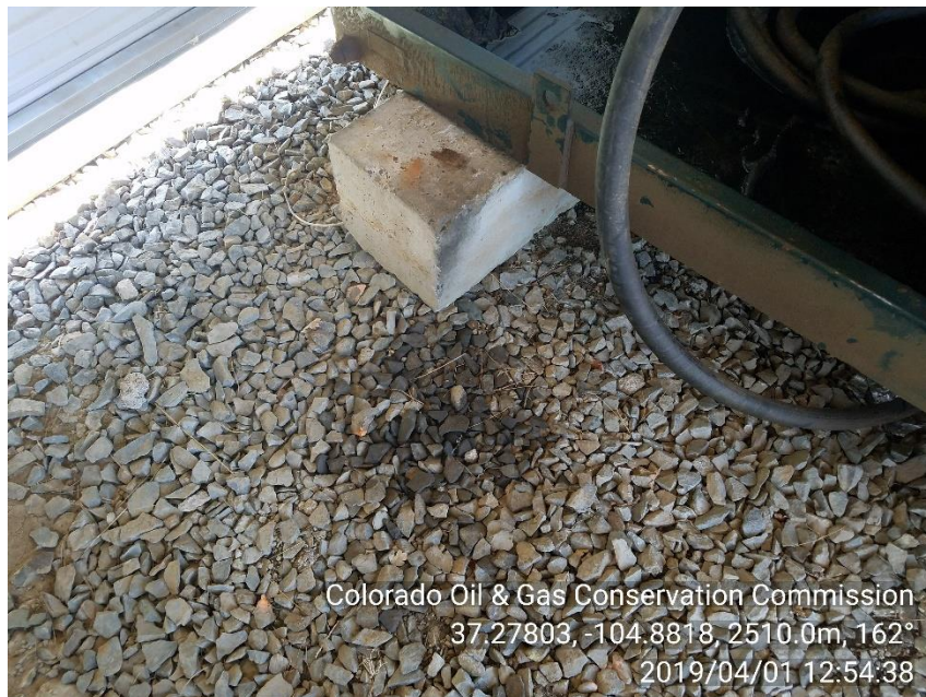
PHOTO 5: IMPACTED SOIL NEAR BACK ( SOUTHEAST) SIDE OF ENGINE SKID
