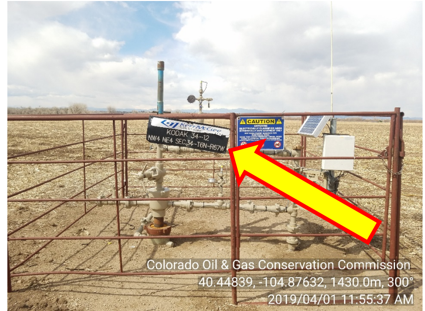
Photo #2 Kodak 34-12 Wellsite Shut-In | SI Emergency Number – Remains NOT Legible
