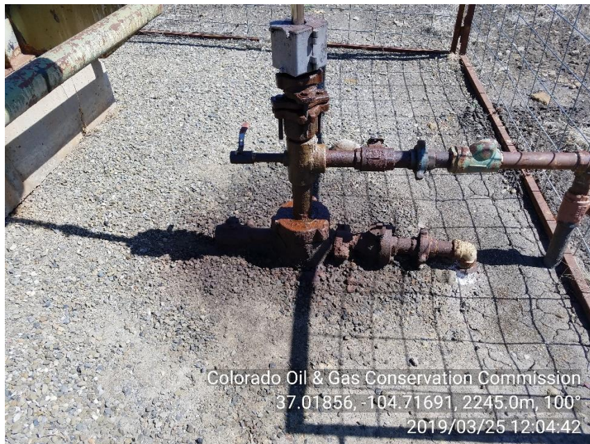
PHOTO 3: WELLHEAD IS COATED WITH A GREASY/ OILY APPEARING SUBSTANCE THAT IS IMPACTING SOIL IN ABOUT A 2' RADIUS AROUND WELLHEAD.
