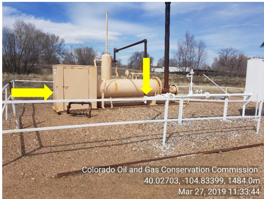
Photo 3 Equipment not anchored
