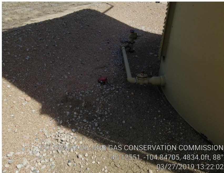
Pic 7 Unused unmarked riser by oil tank
