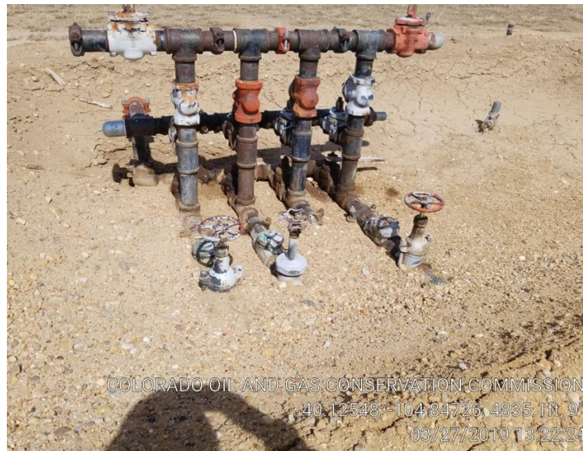
Pic 8 manifold with stained soil.
